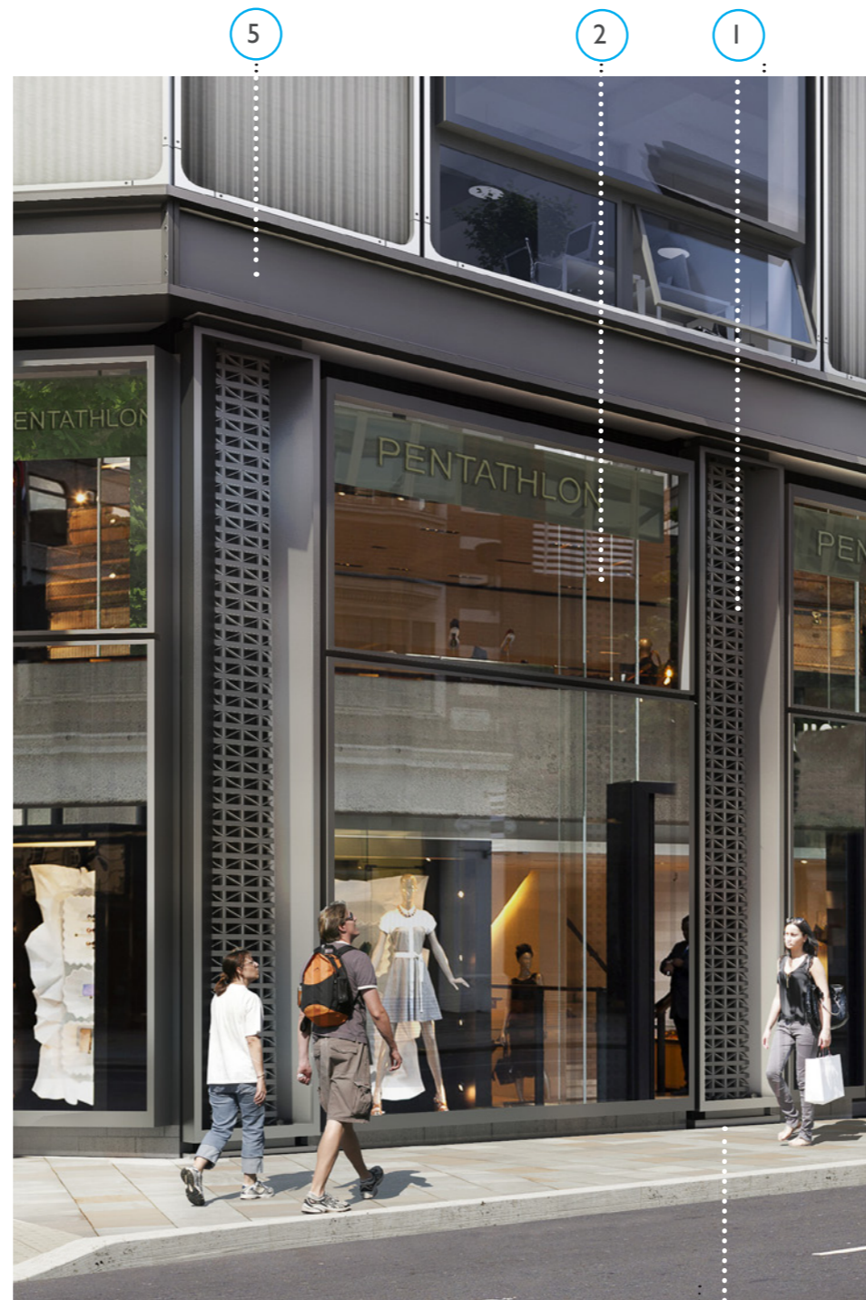
View of south west corner from High Holborn showing public use
