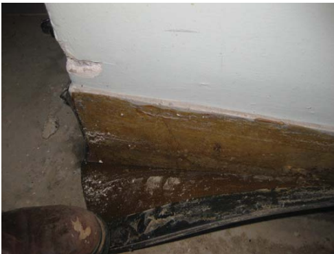
existing terrazzo with vinyl sheet and sheet adhesive. All to be replaced
