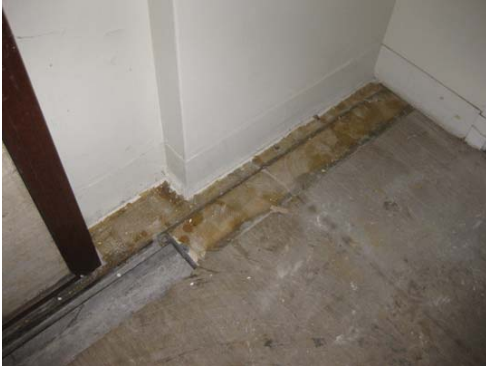
existing terrazzo with vinyl sheet and sheet adhesive. All to be replaced
