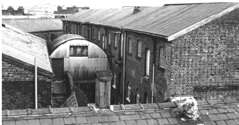
Figure 5 Provender Store: northwest corner in 1976
