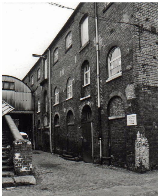
Figure 4 1976 Photograph of Provender Store north elevation
