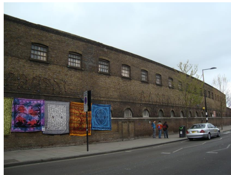
Figure 3 The 'Camden Wall', Chalk Farm Road.
