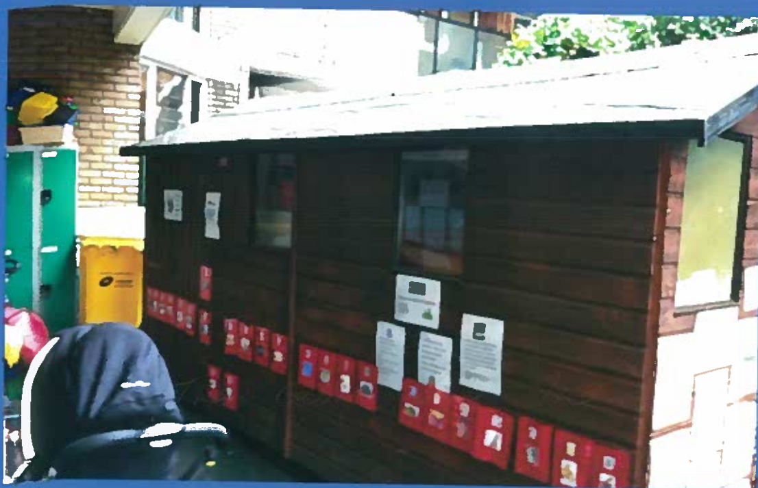
The old sheds - 1 large unit with windows 2 doors lights and plug sockets for equipment
