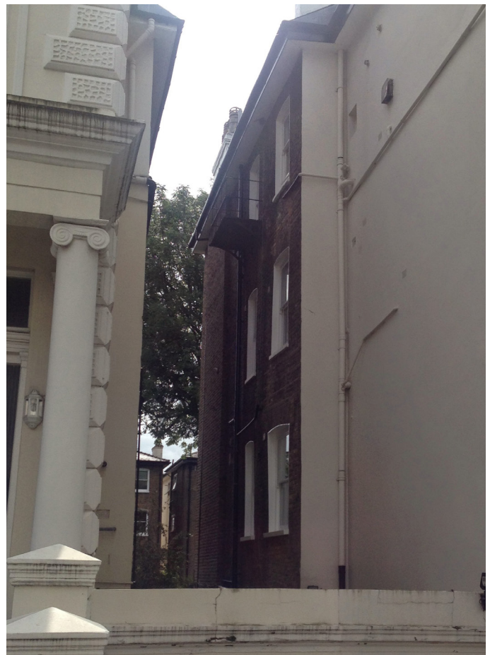
View of the side facade to No. 15 Belsize Park Gardens
