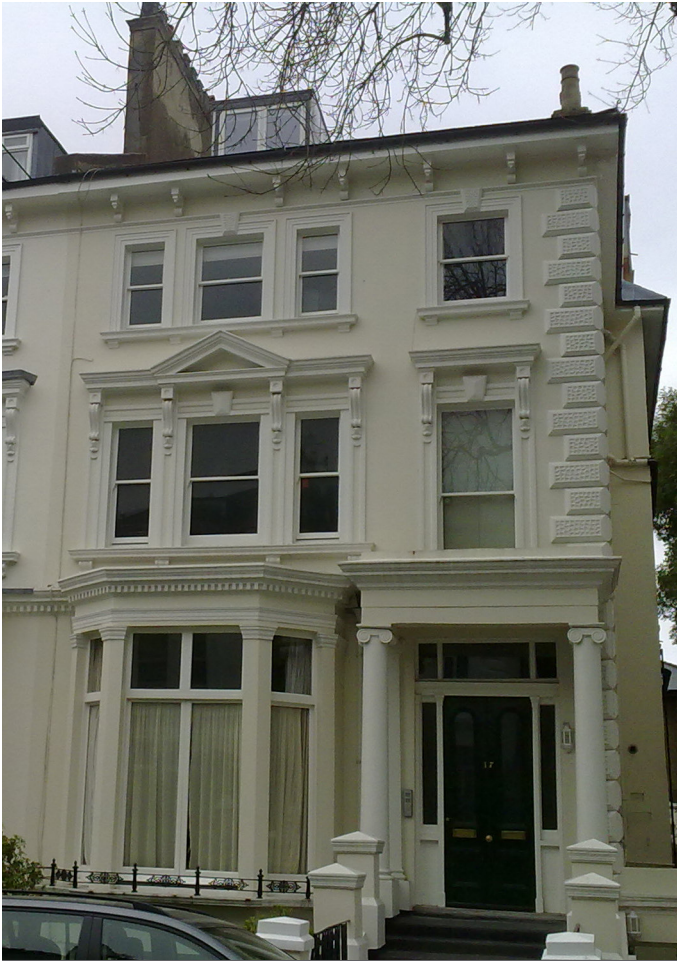
View of the front facade of 17 Belsize Park Gardens
