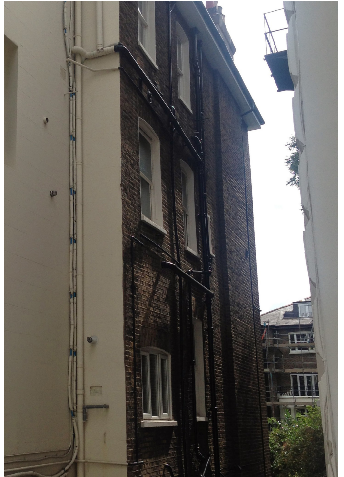
View of the side facade of 17 Belsize Park Gardens
