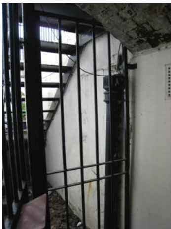
basement flat metal security gate
