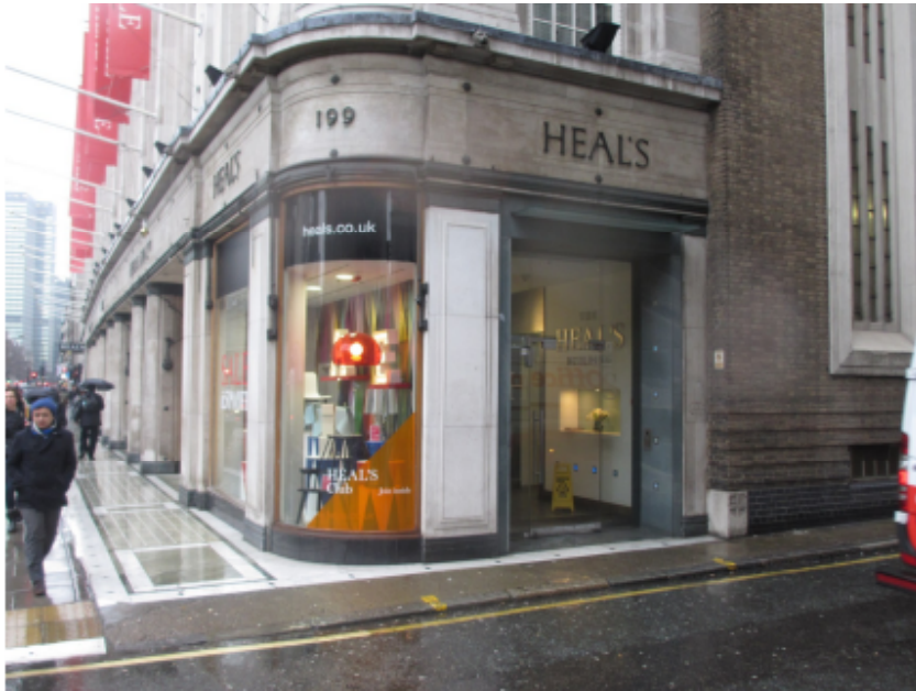
Existing Office entrance on Alfrew Mews
