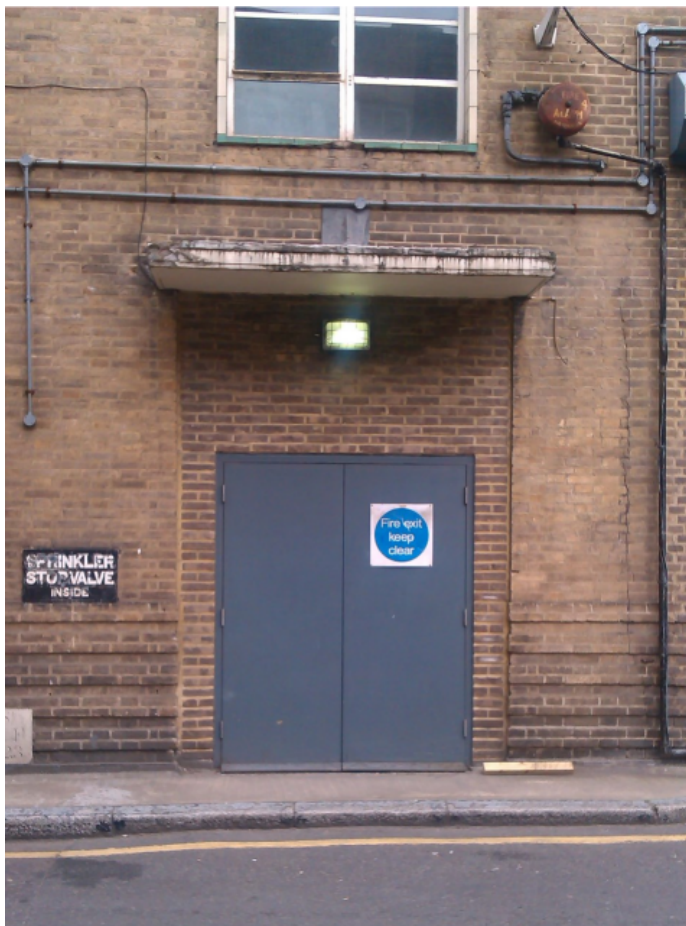
Existing Service entrance on Alfred Mews
