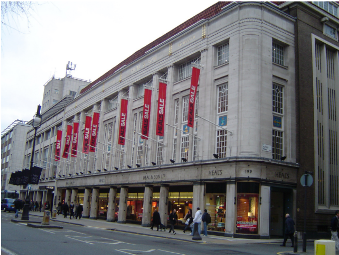
Existing Heal's frontage on Tottenham Court Road
