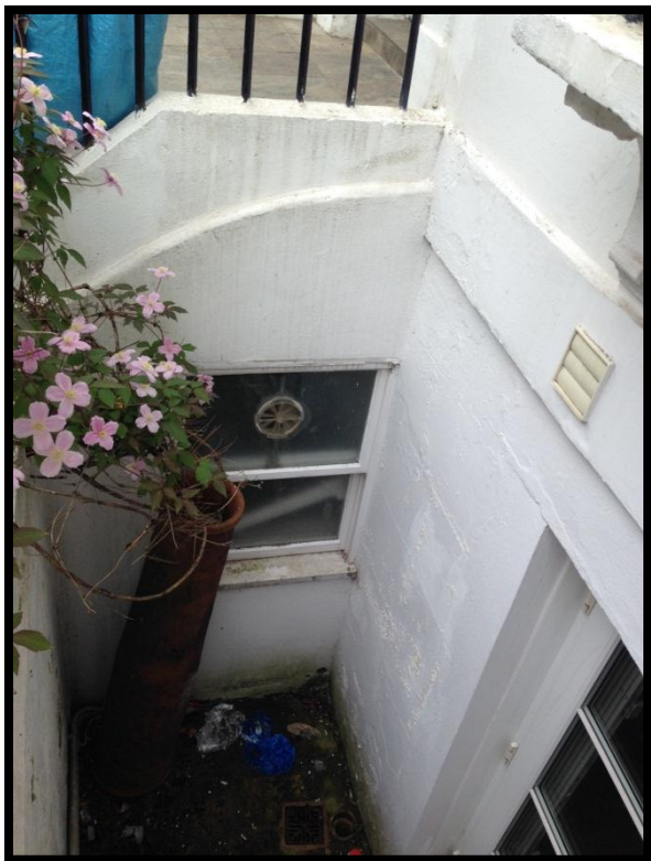
Photo 3: Bathroom window to be replaced with timber window.
