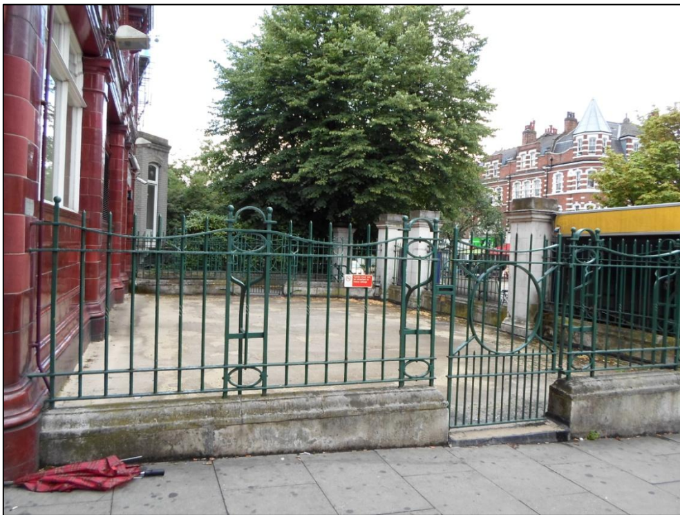
Figure 2: Photograph showing the forecourt at the front of Belsize Road station where the new manhole inlet is proposed.
