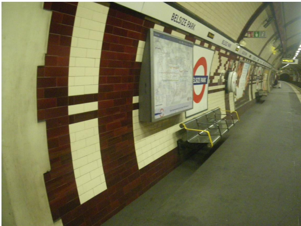
Figure 8: Photograph showing location of new dry riser outlet cabinet to be located on Platform 1 (see drawing TLL-L001-FUNC-FIR-DRW-00070)
