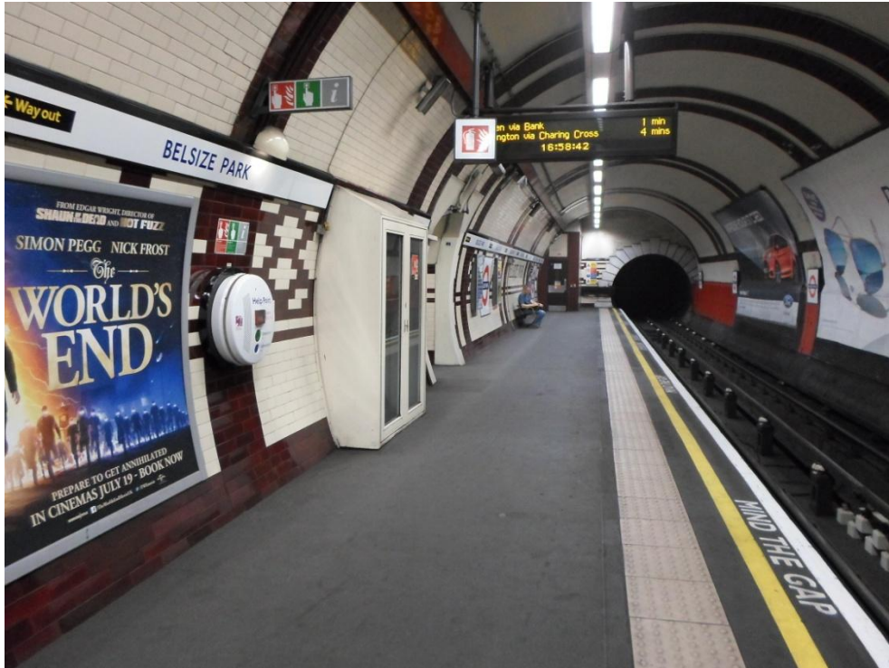
Figure 7: Photograph showing the existing hydrant outlet cabinet on platform 2
