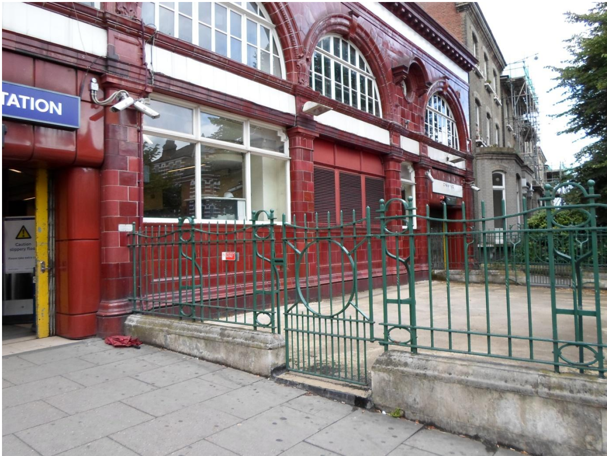
Figure 1: Photograph of the facade of the Caledonian Road Station illustrating that the addition of the inlet box flush with the forecourt at this location will be insignificant in effect to the heritage significance of the Leslie Green facade.
