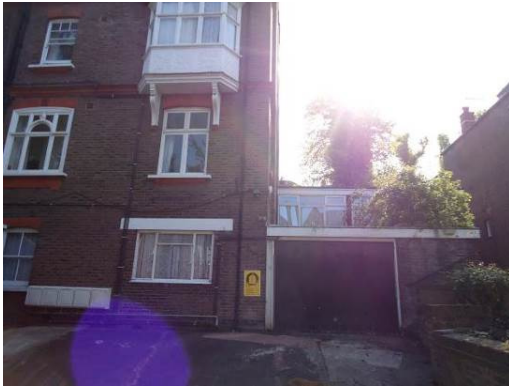
Side extension and garage
