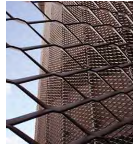
Anodised aluminium 'Eye-tech' expanded metal screen over brick cladding
