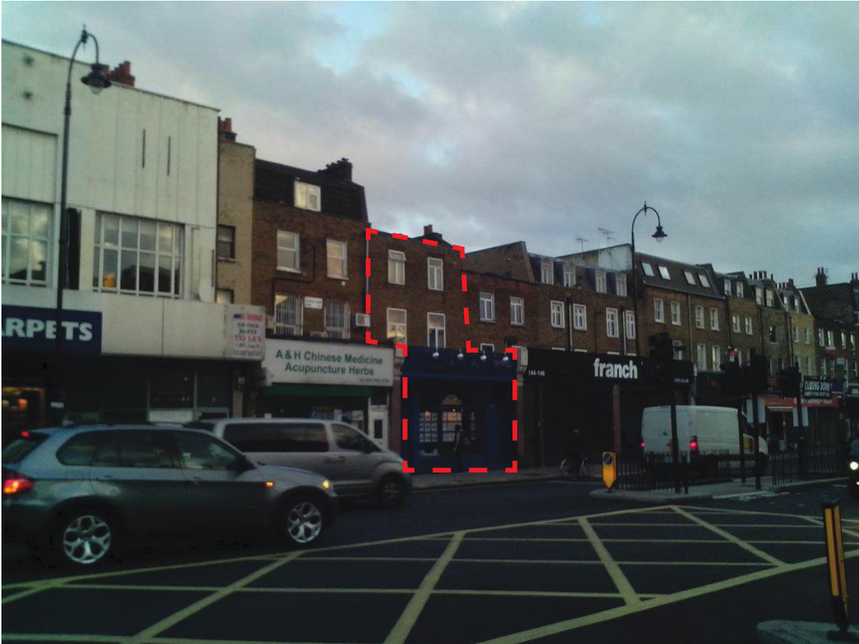
Fig 2: View of site from Prince of Wales Road
