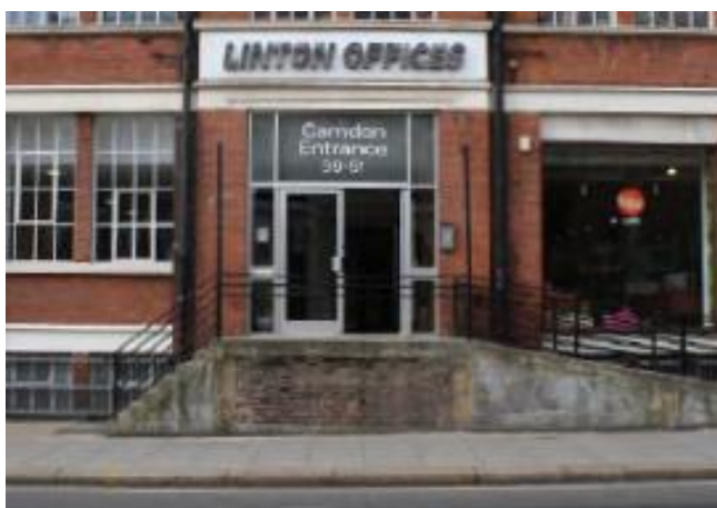
Figure 2: Current Main Entrance to Linton House
