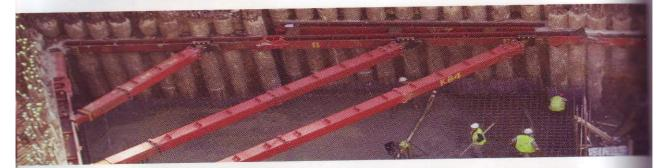
The MGF 400 Series Hydraulic Strut System is capable of spanning up to 24m without any intermediate support and is fully compatible with the MGF 406 Waler System and MGF 1250kN and 2500kN Modular Components. This system is primarily used to support RC capping beams as well as modular and bespoke steel / concrete waler systems. This system can be used in both horizontal and raking applications to support excavations / structures.
