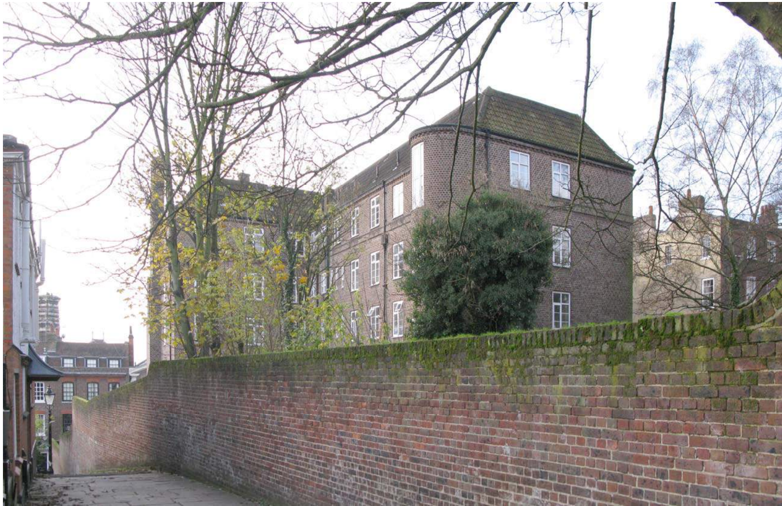
Existing view from Christchurch Passage
