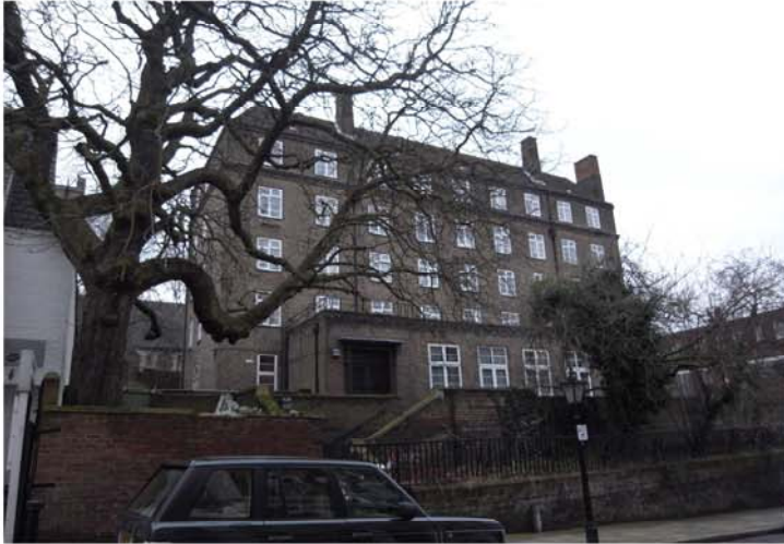
PHOTOGRAPH - EXISTING BUILDING
