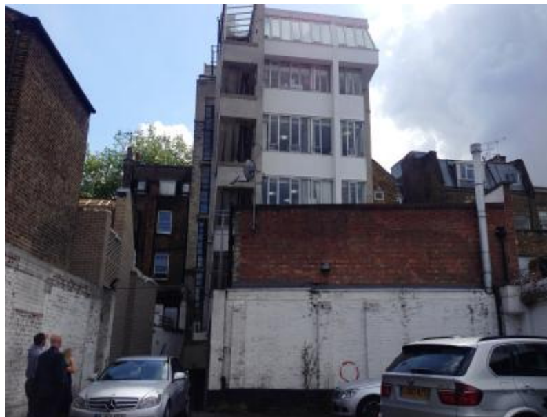
Image 3: Side of view of site
