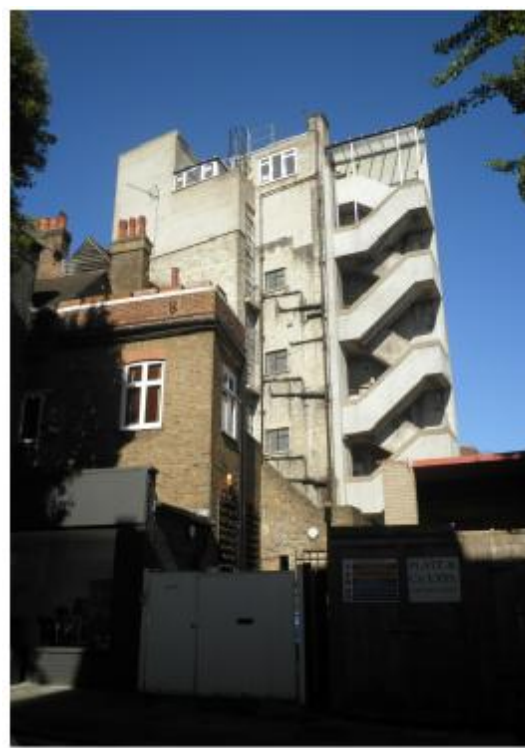
Image 5: View of Rear Fire Escape
