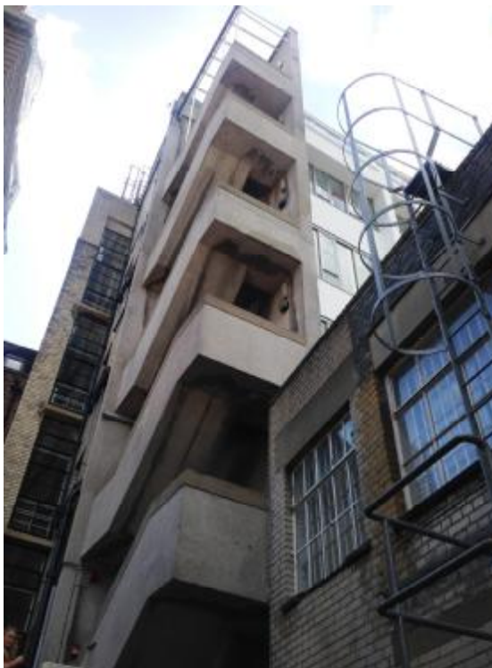
Image 4: View of Rear Fire Escape
