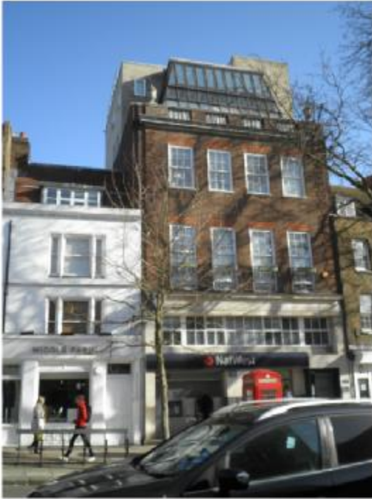
Image 1: View from Hampstead High Street of site
