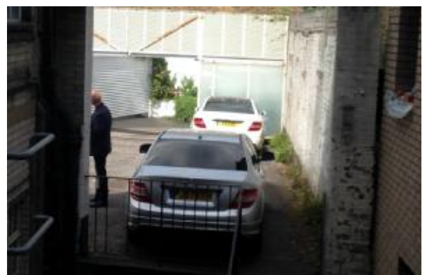
Image 7: View of existing fence and gate
