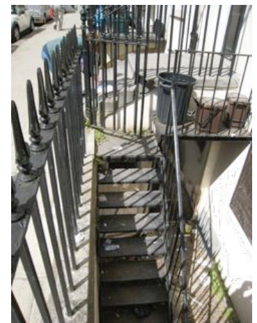
basement flat entrance
