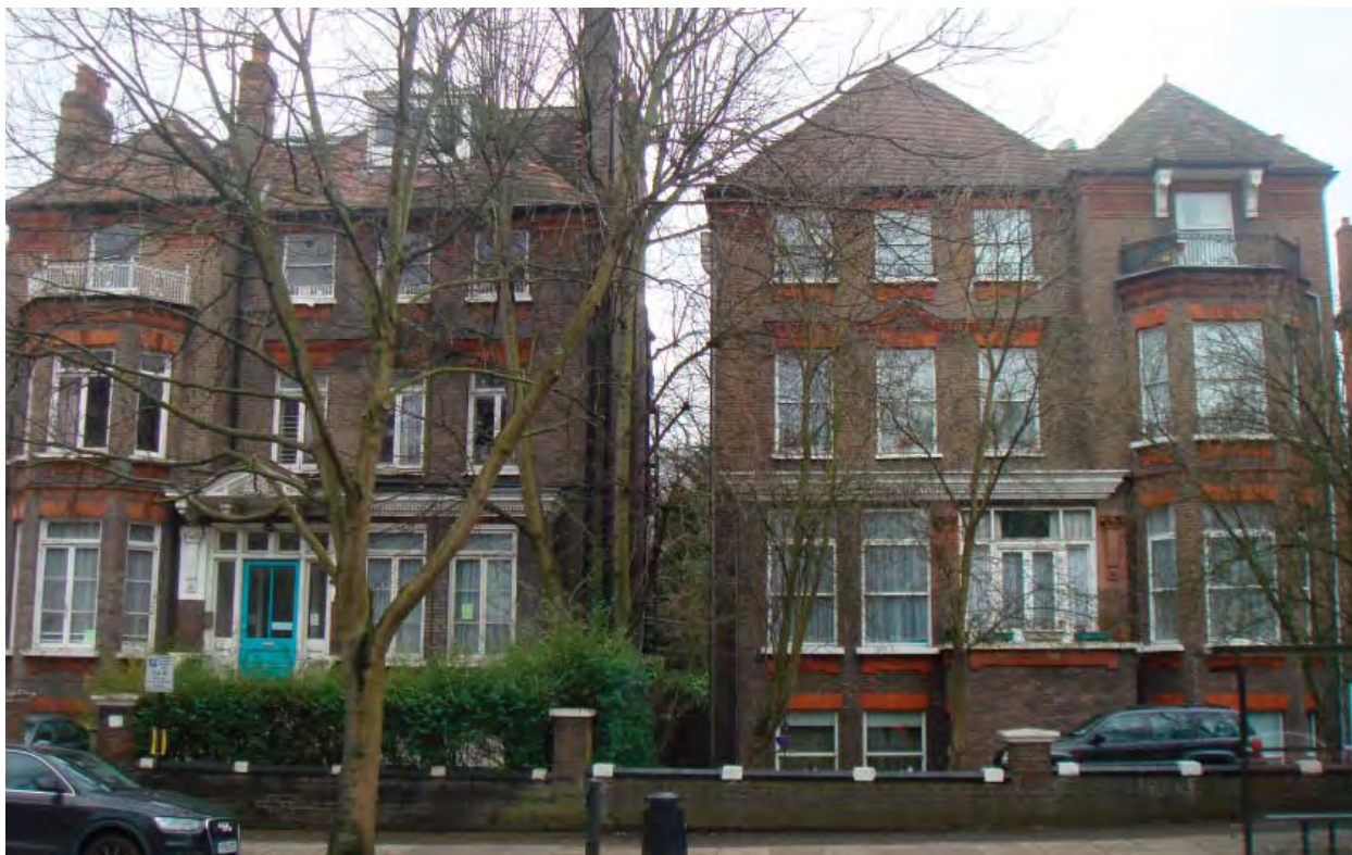
Fitzjohn's Avenue - paired villas with similar facade structure to the no.2 Maresfield Gardens
