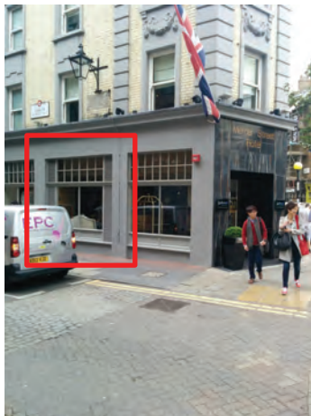
Mercer Street Hotel – Radison Blu
