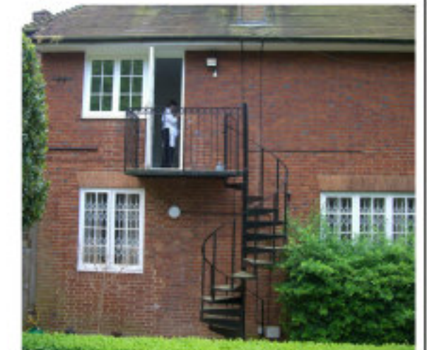
EXISTING BALCONY- IMAGE 01
