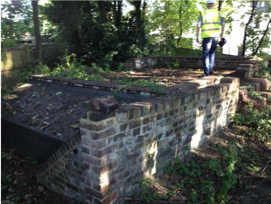
Fig. 5: Existing Garage with raised roof terrace & steps.
