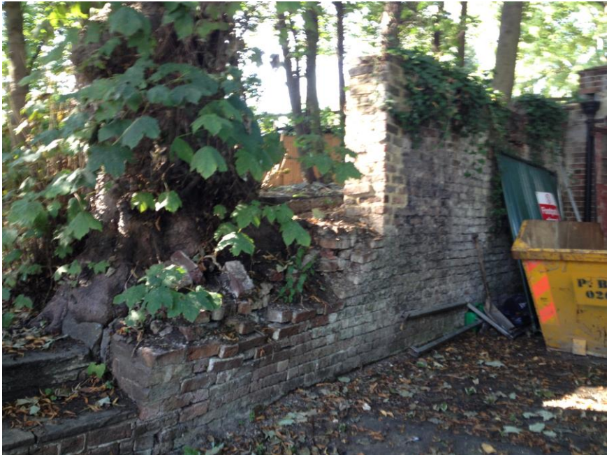
Fig. 4: Brick wall along southern edge of Garage.
