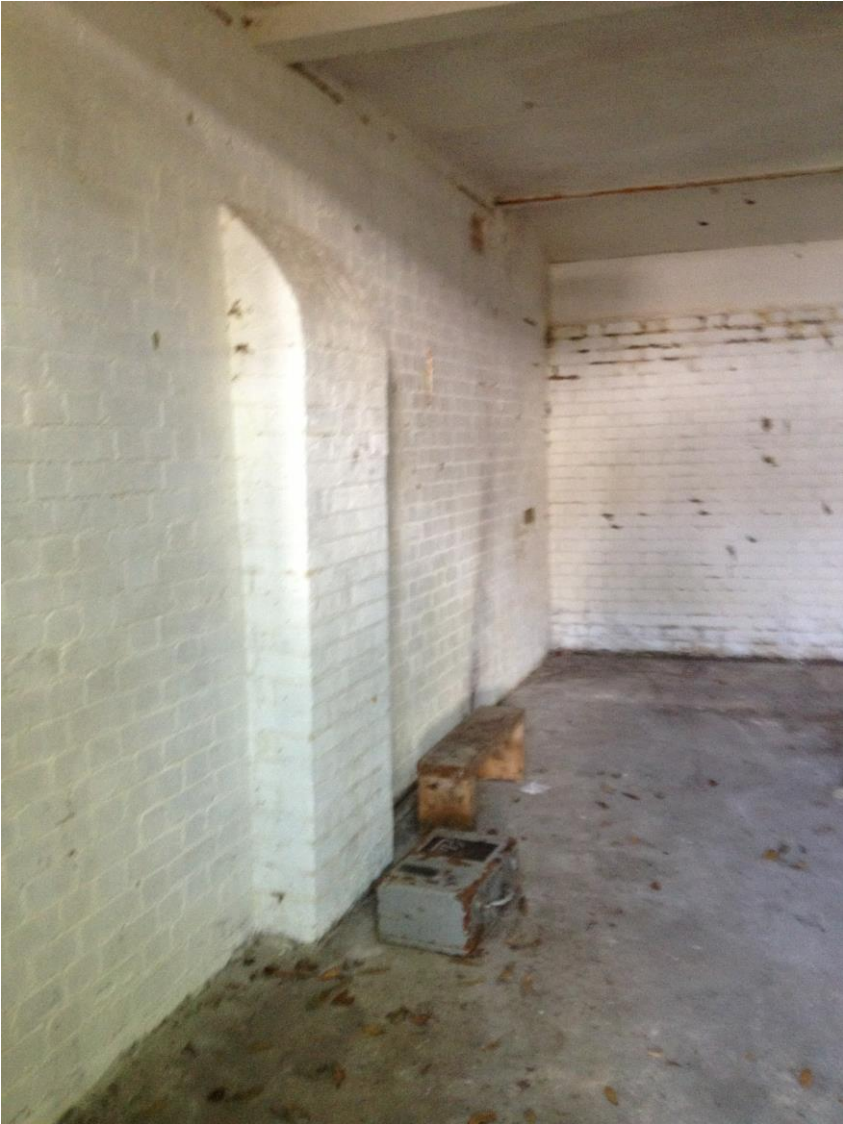
Fig. 6: Garage Interior in 2013.
