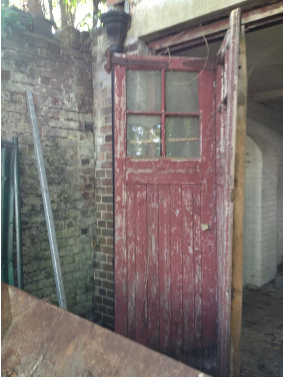
Fig. 7: Garage entrance doors in 2013.
