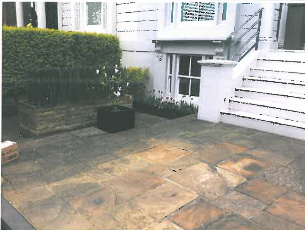
Photo 3 – View of front drive. Note stepped terracing of paving to left hand side of front door, and light well at front window.
