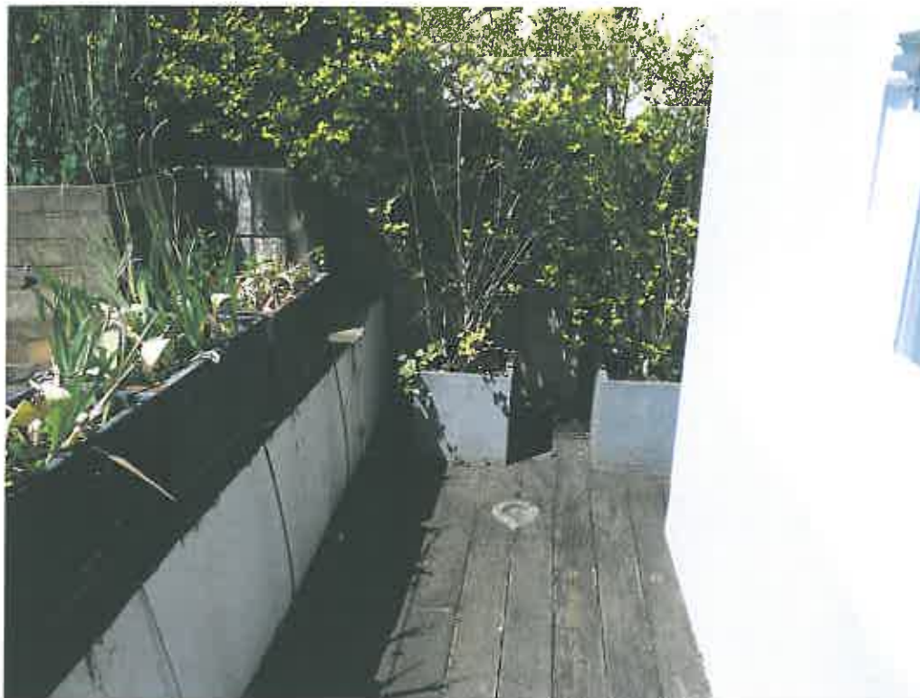
Photo – Detailed view of light well at front of house
