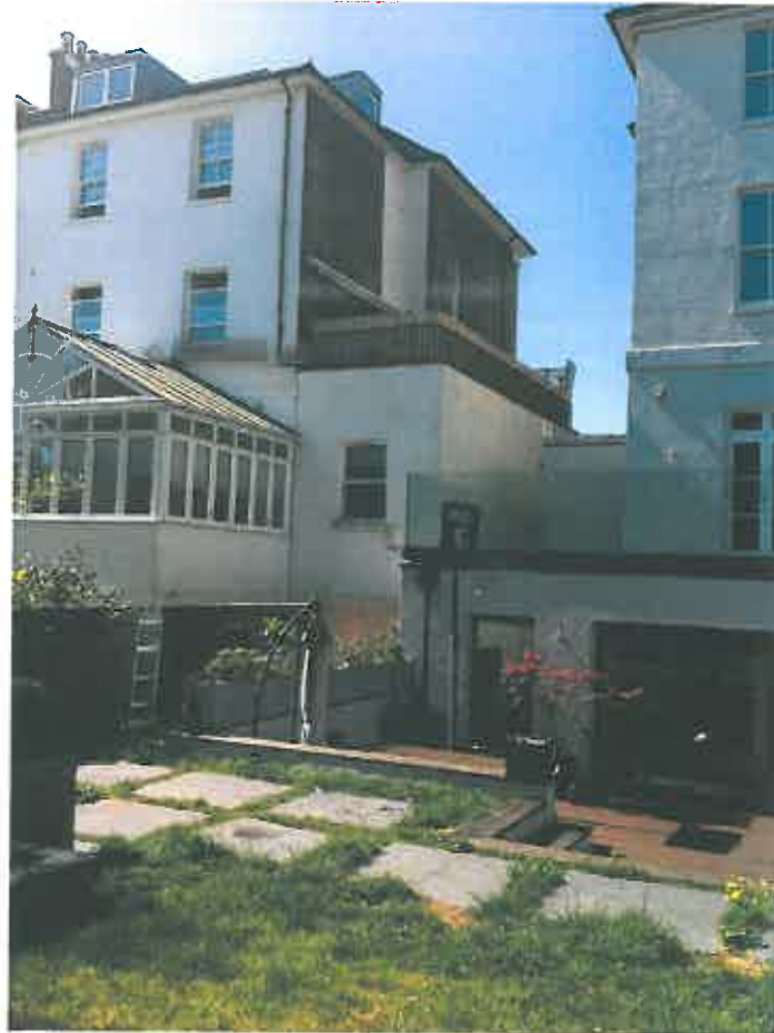
Photo 5 – View from rear garden of terrace at rear of ground floor.
