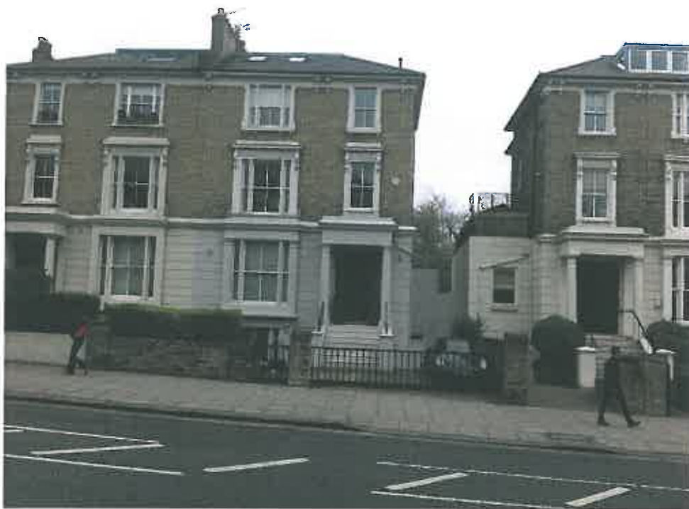
Photo 1 – General View of front of house (centre frame) from Haverstock Hill. Note general slope of Haverstock Hill from left to right, towards south east.
