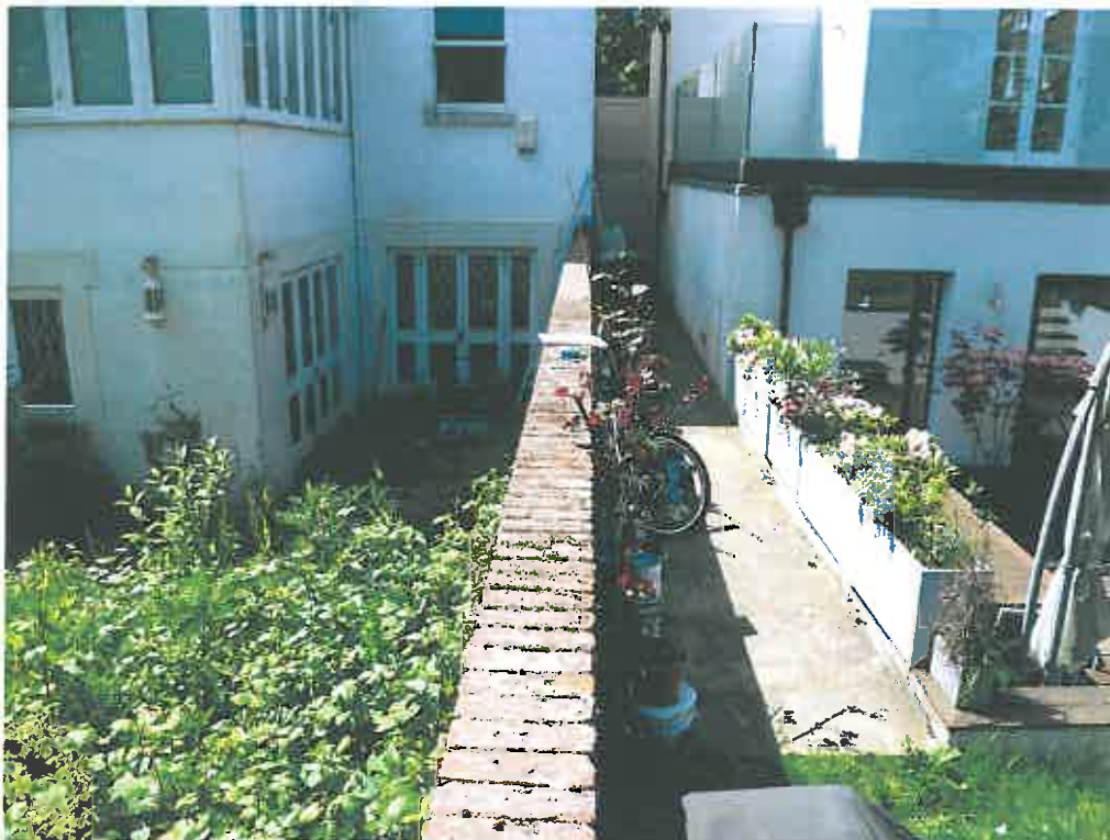
Photo - View of 166/168 boundary and side passage.
