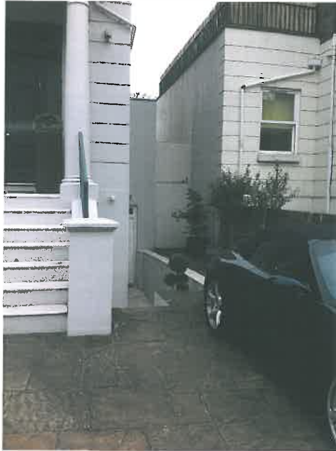
Photo 2 – View along side passage between No168 (left) and No166 Haverstock Hill Note side passage with gated access to rear of house, and reduced level passage to gain access to ground floor. Steps on left rise to gain access to existing first floor.
