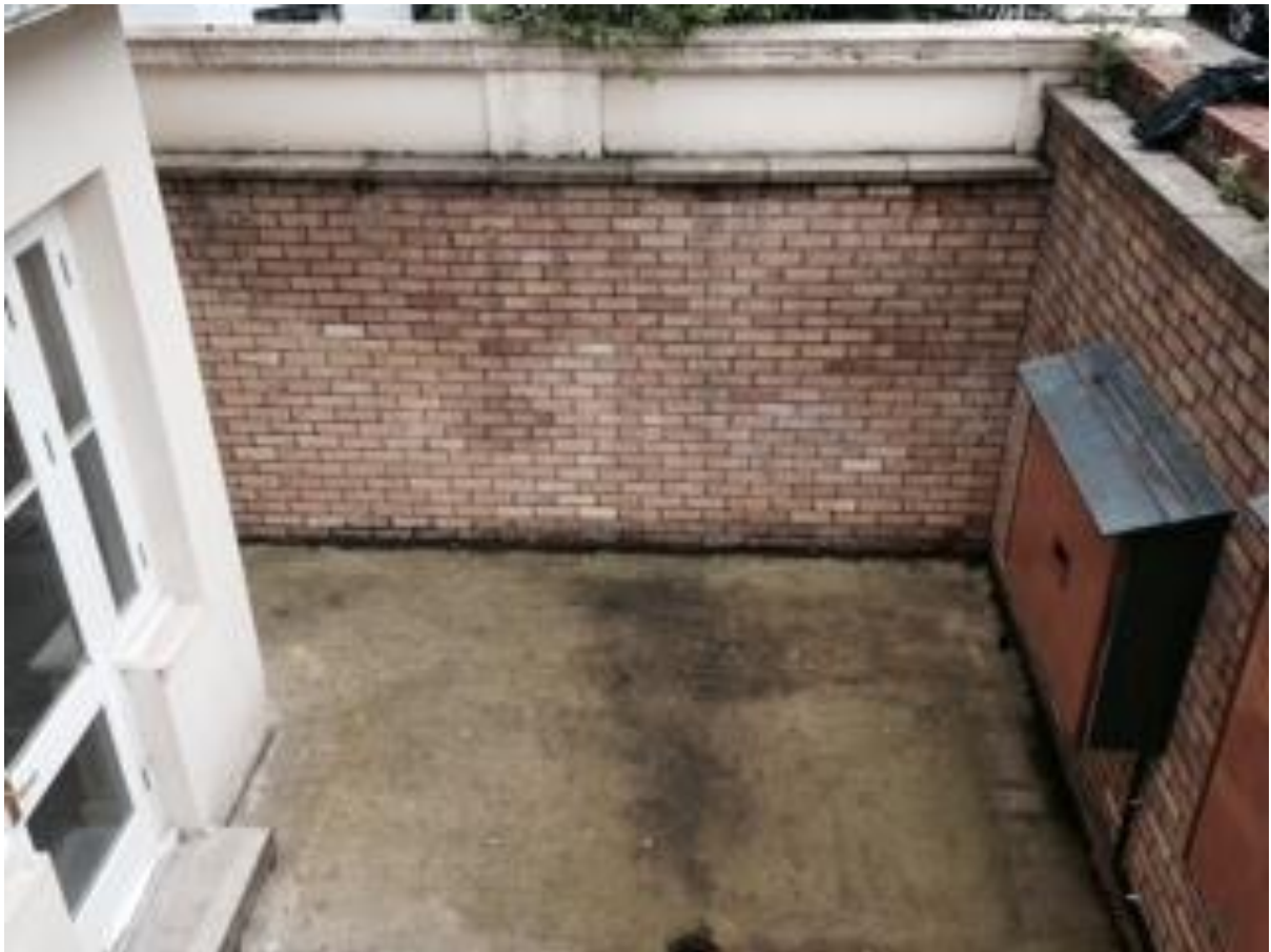
Top: Photo of unauthorised door installed in place of window.
