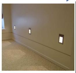
Recessed low level LED interior wash light with low-glare asymmetrical reflector
