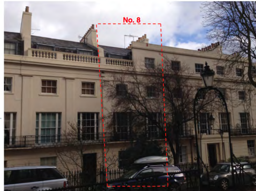
Photograph of the central portion of the terrace, viewed from Chester Place
