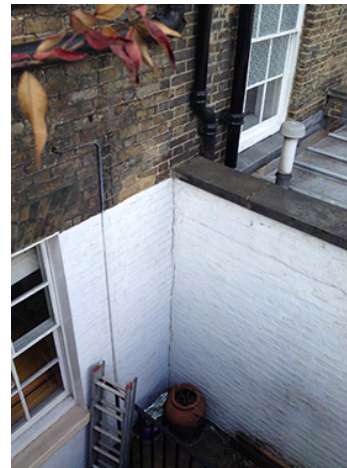
External rear courtyard
