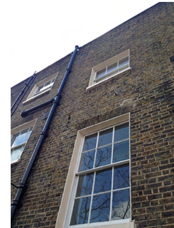
Rear single glazed sash windows
