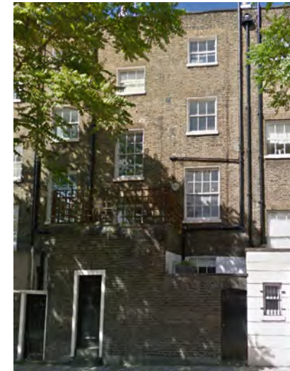
Brick façade facing onto Albany Street
