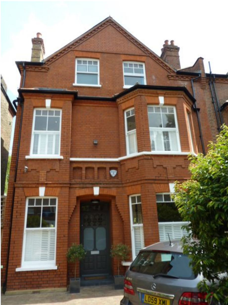
the front facade
