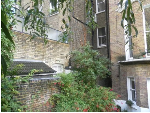
(5) Party wall between 26 & 28 Fellows Road
