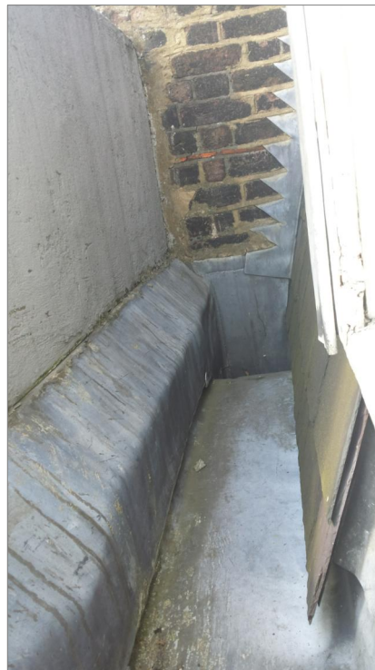
IMAGE OF EXISTING GUTTER
