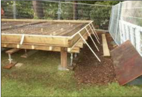
Photo 36: Small diameter piles (less than 150mm) are an effective means of supporting structures in RPAs with minimal disturbance.
