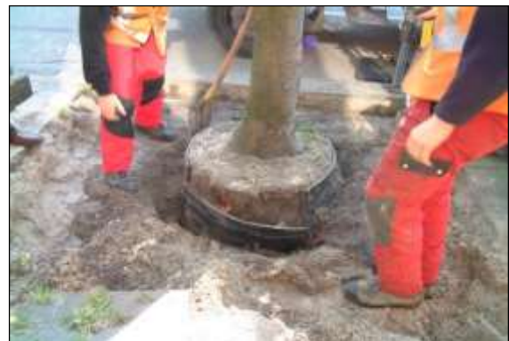
Photo 58: This excavated tree shows the root deflectors that were installed when it was planted seven years previously. The product has deflected roots downwards and prevented damage to the adjacent surfacing. Note that this is a permeable sandy soil and the roots were able to grow beneath the bottom of the deflectors.
