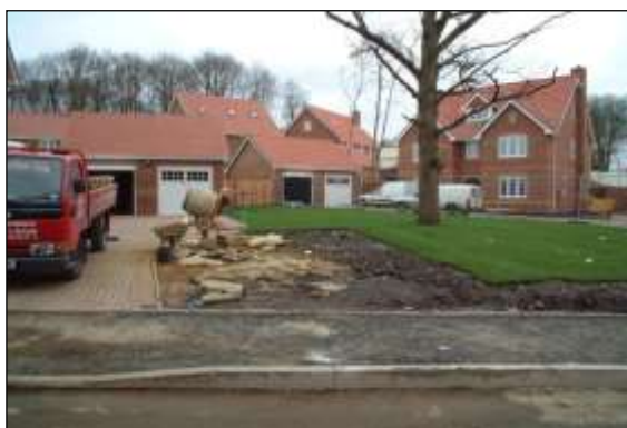
Photo 48: The RPA of this tree was not effectively protected during construction and excessive compaction of the soil meant it died soon after this turf covered up the damage.
