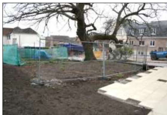
Photo 49: This tree had tarmac parking within its RPA that was removed and replaced with an organic mulch near the trunk and limited no-dig surfacing on the outer edges of its RPA.
