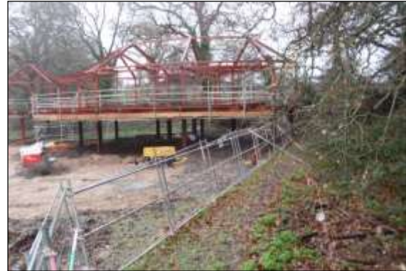
Photo 37: It is possible to support very large structures on piles within sensitive RPAs without any significant adverse impact on tree roots.
