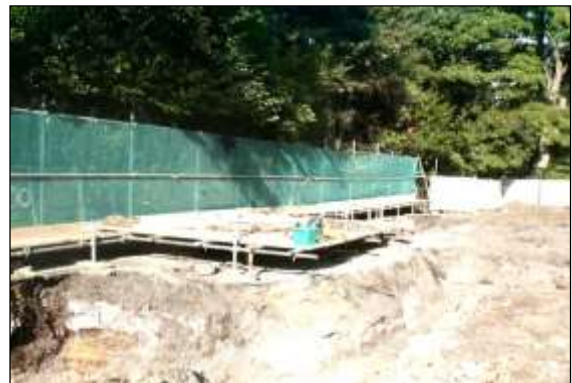
Photo 10: A scaffold framework attached to the main scaffold fencing can be used to support either scaffold planks or plywood to create an elevated platform with a gap beneath.
