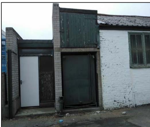
Photograph showing green coloured metal tank containing hydrocarbon
