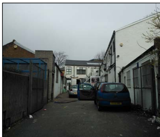
Photograph showing general arrangement of the site, looking northeast from access road
