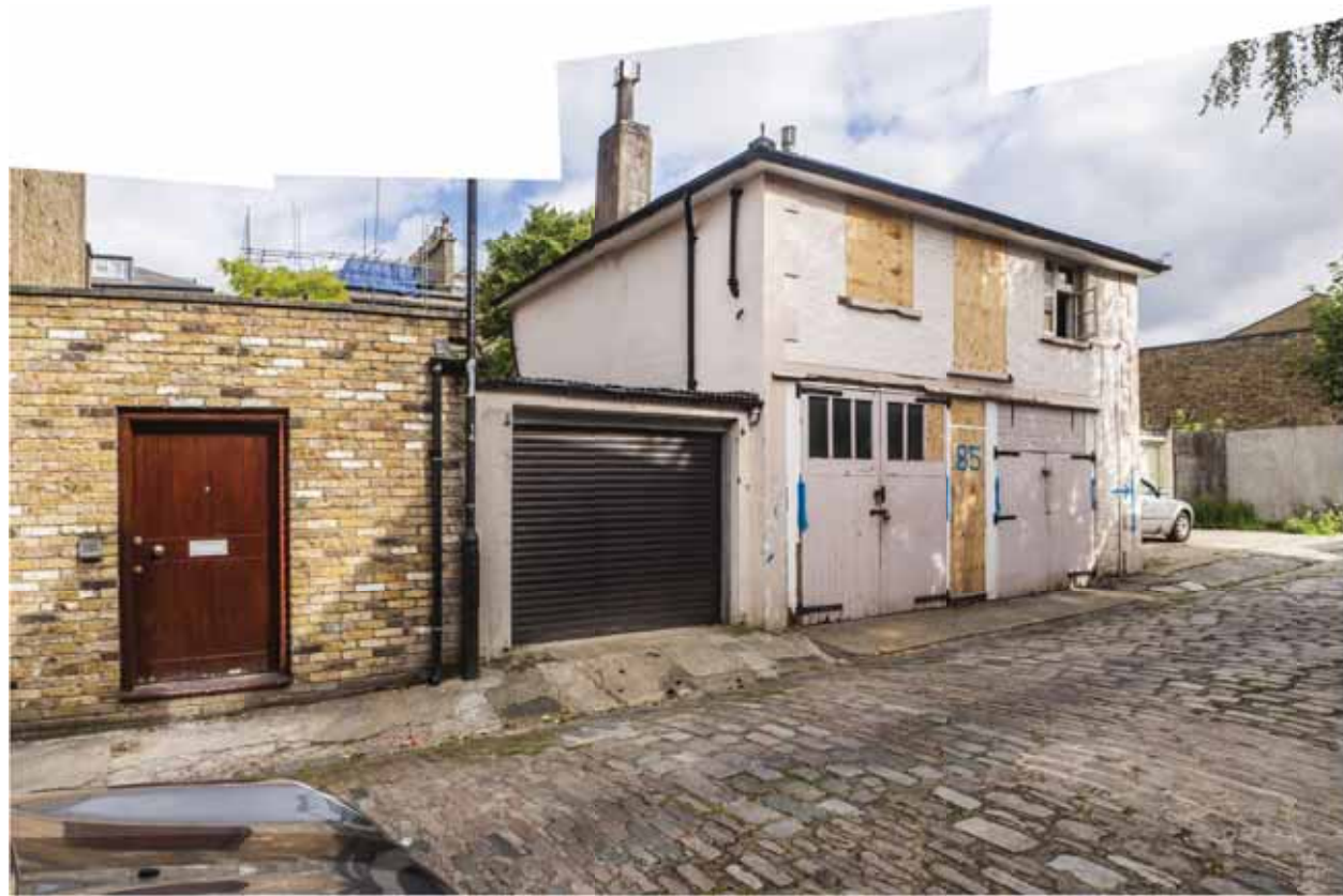
A View of South East Facade Garage to be replaced
