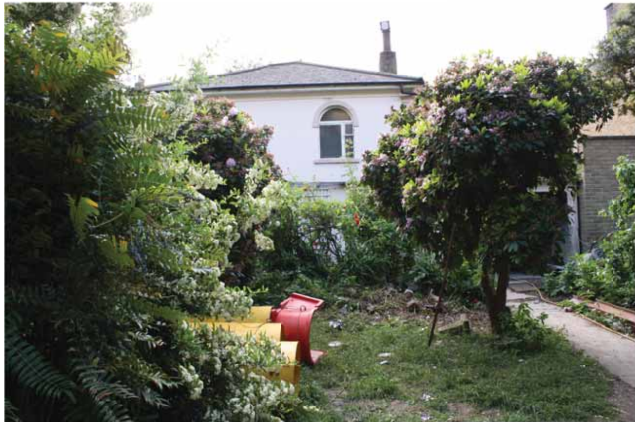
C View of North West Facade through garden
