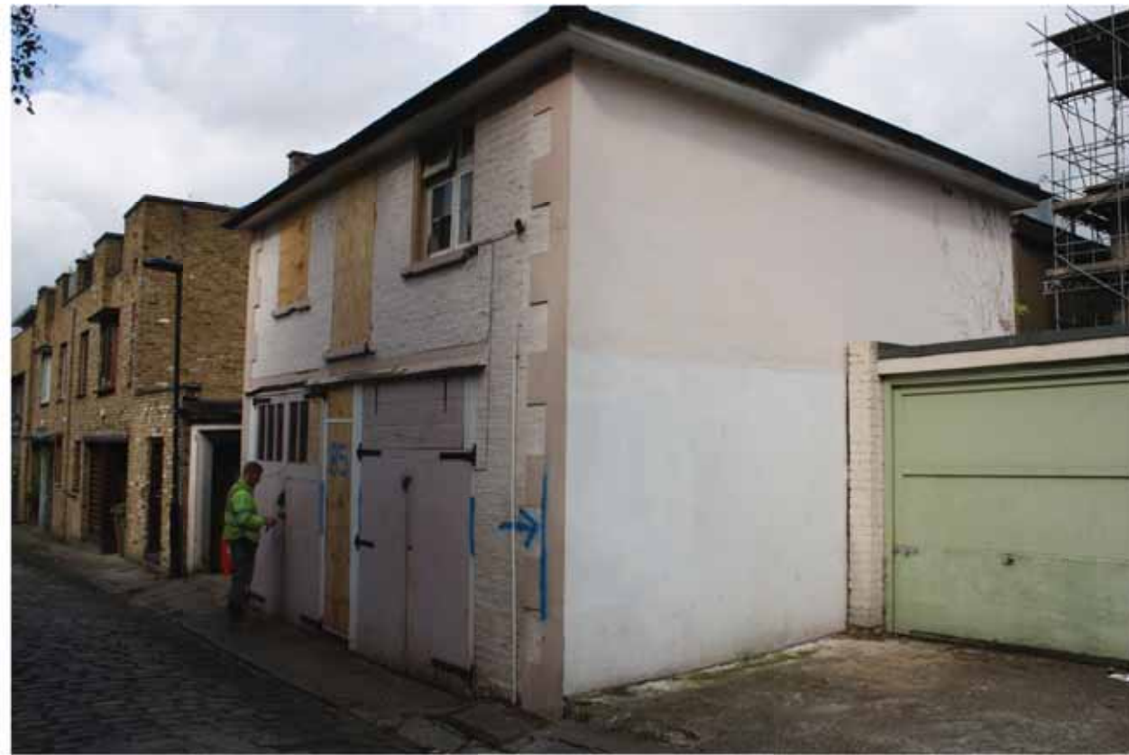
B View of South East Facade
