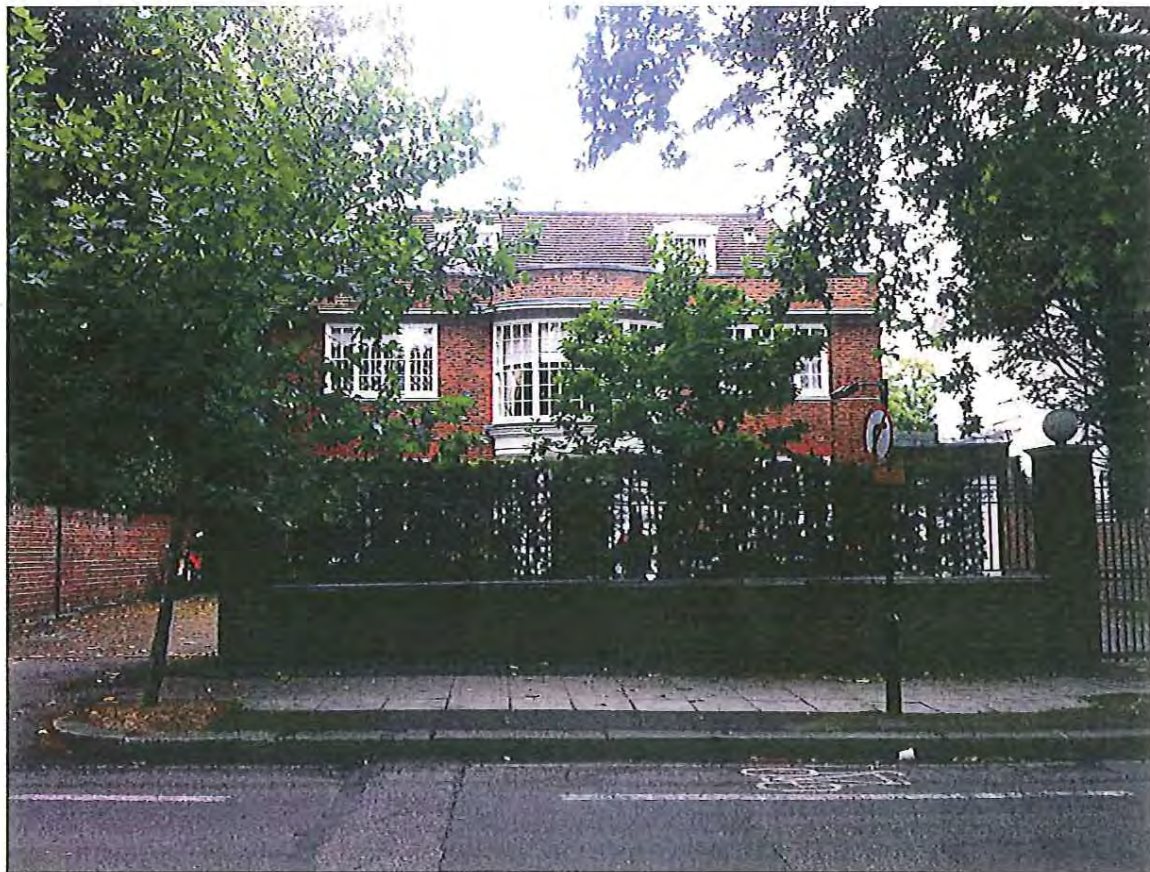
Photo 1- The property as viewed from Avenue Road
