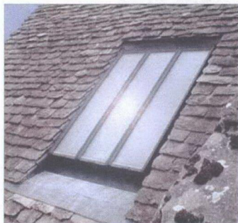
Flush fitting, glazing bars, slim sections and stepped glazing detail on the bottom edge give the appearance of a single glazed traditional unit.
