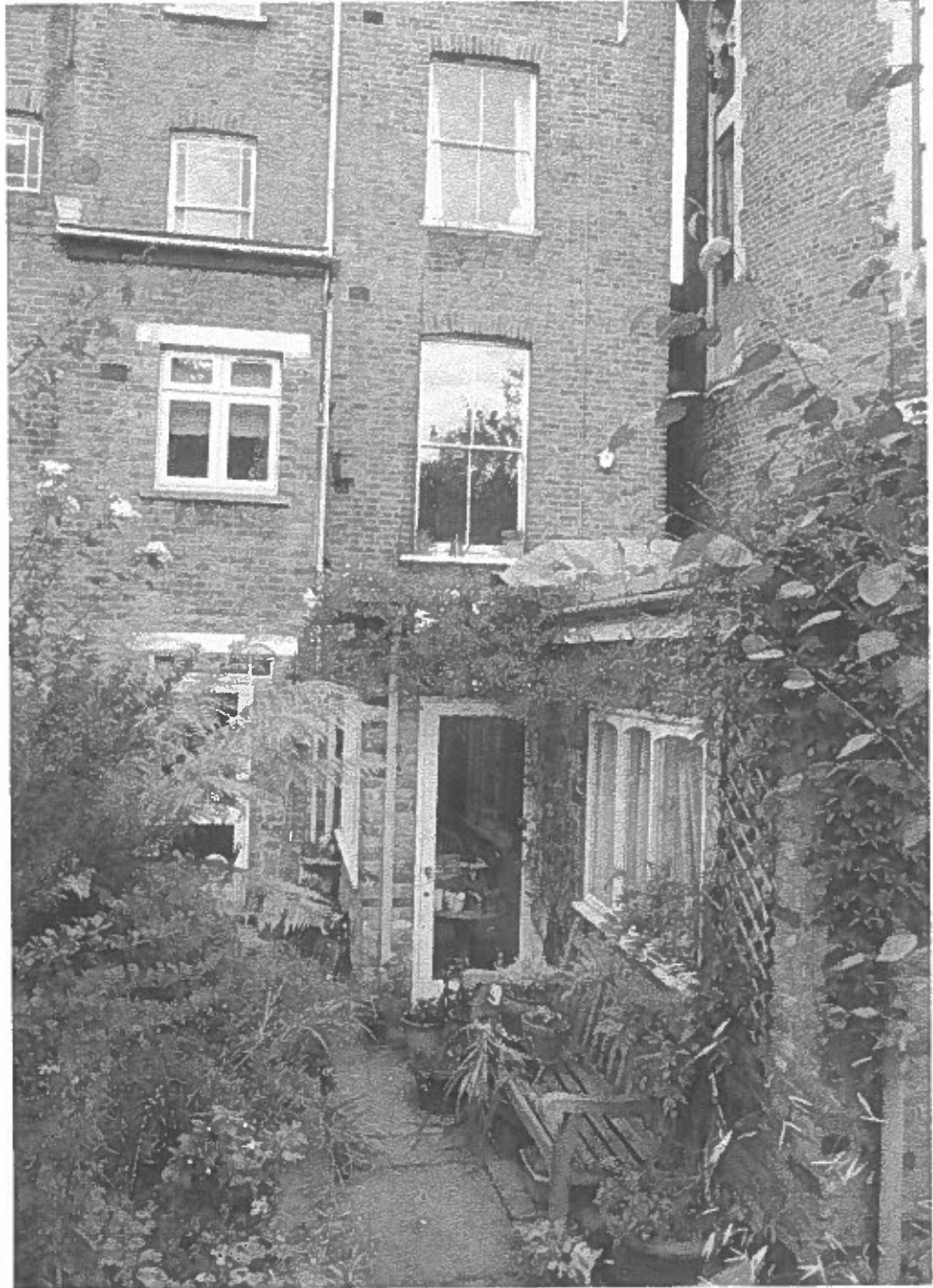
22A North Villas rear extension to house.
