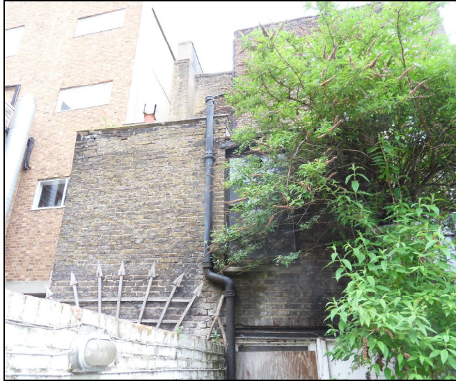
BACK EXTENSION REAR WALL - UPPER STOREY
