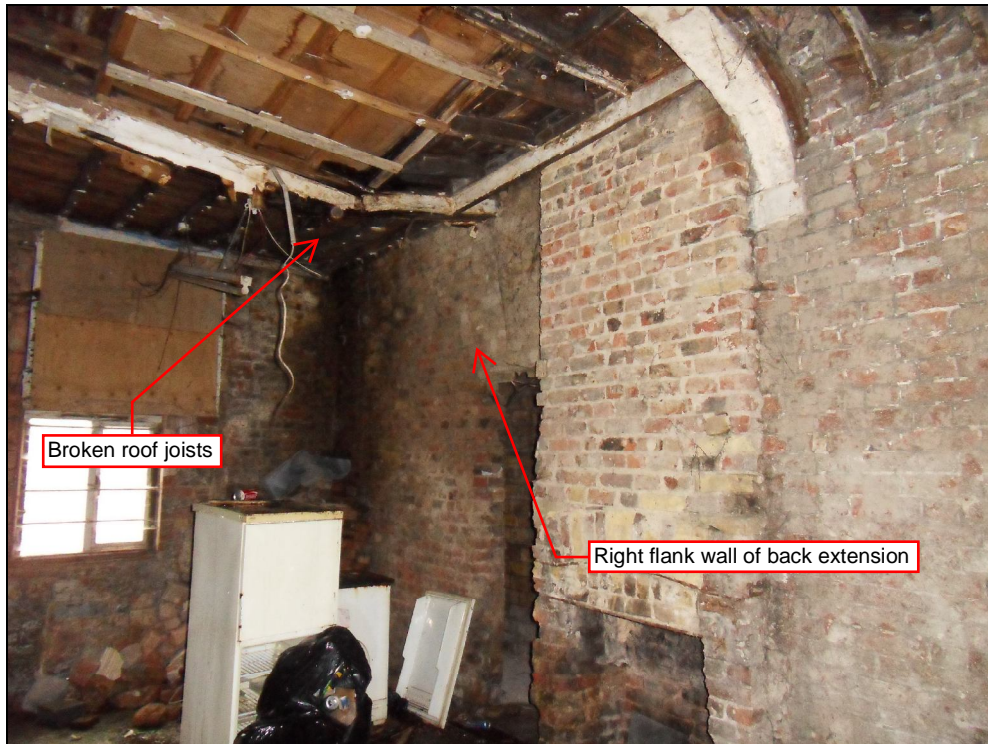
INTERNAL VIEW IN SINGLE STOREY ADDITION – VIEW TO REAR
