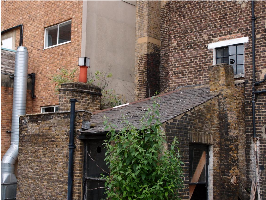
Figure 7 – Rear extension return wall & Chimney
