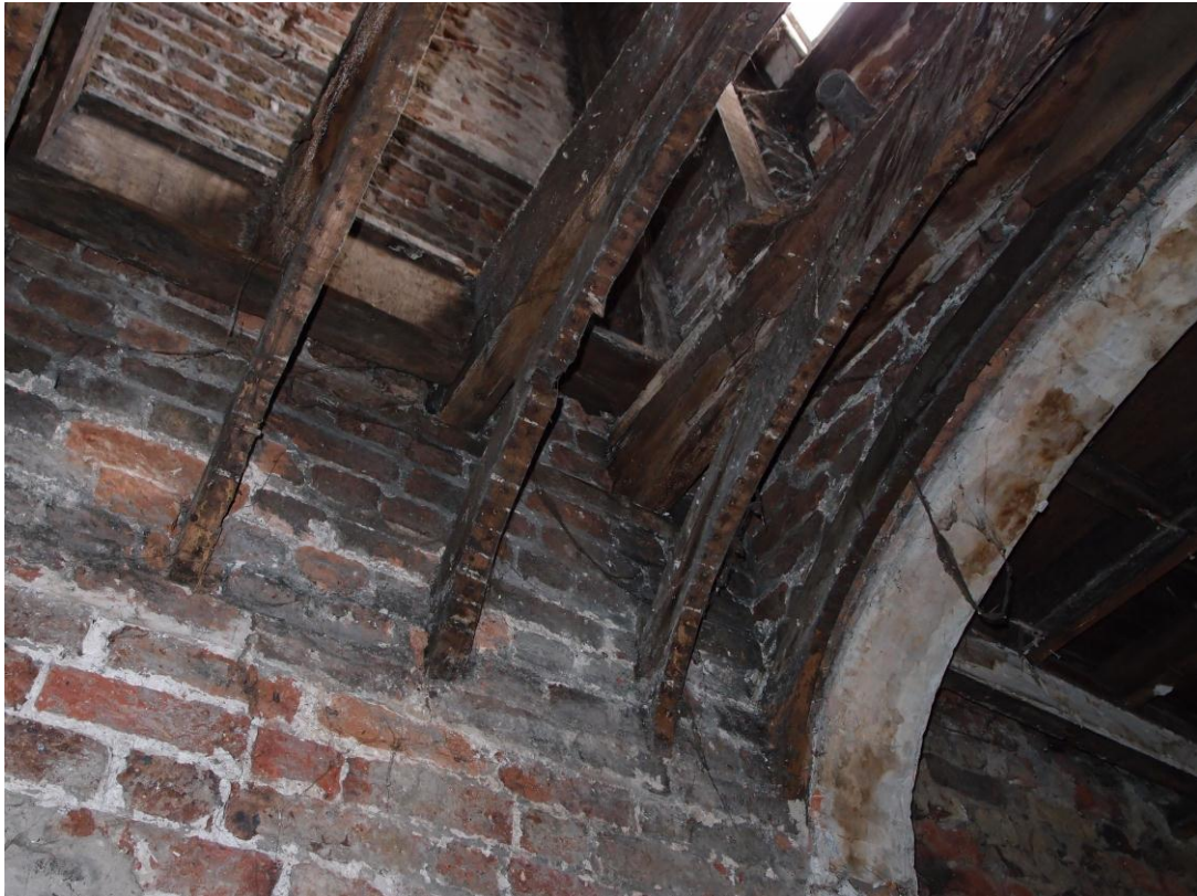
Figure 23 – Rear courtyard entrance first floor joists with arch formers
