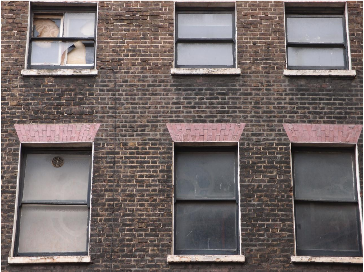
Figure 26 – Typical wooden sash window and stone concrete cills
