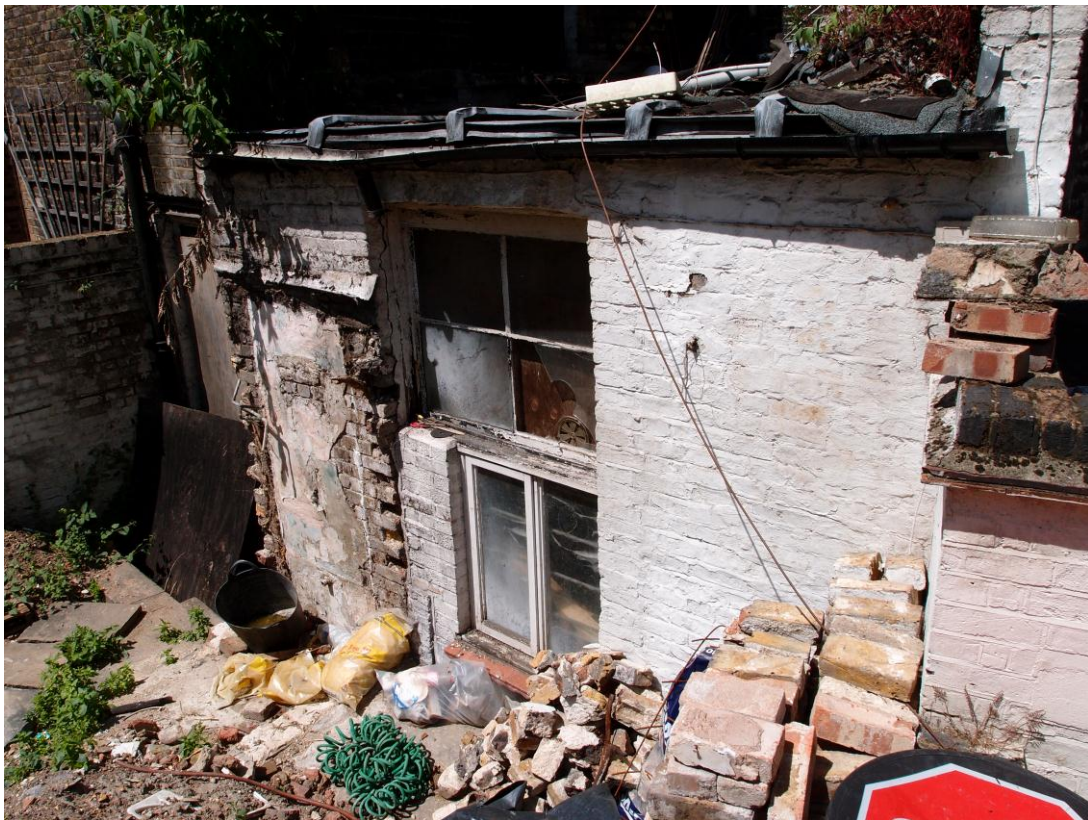
Figure 8 – Rear ground floor external wall
