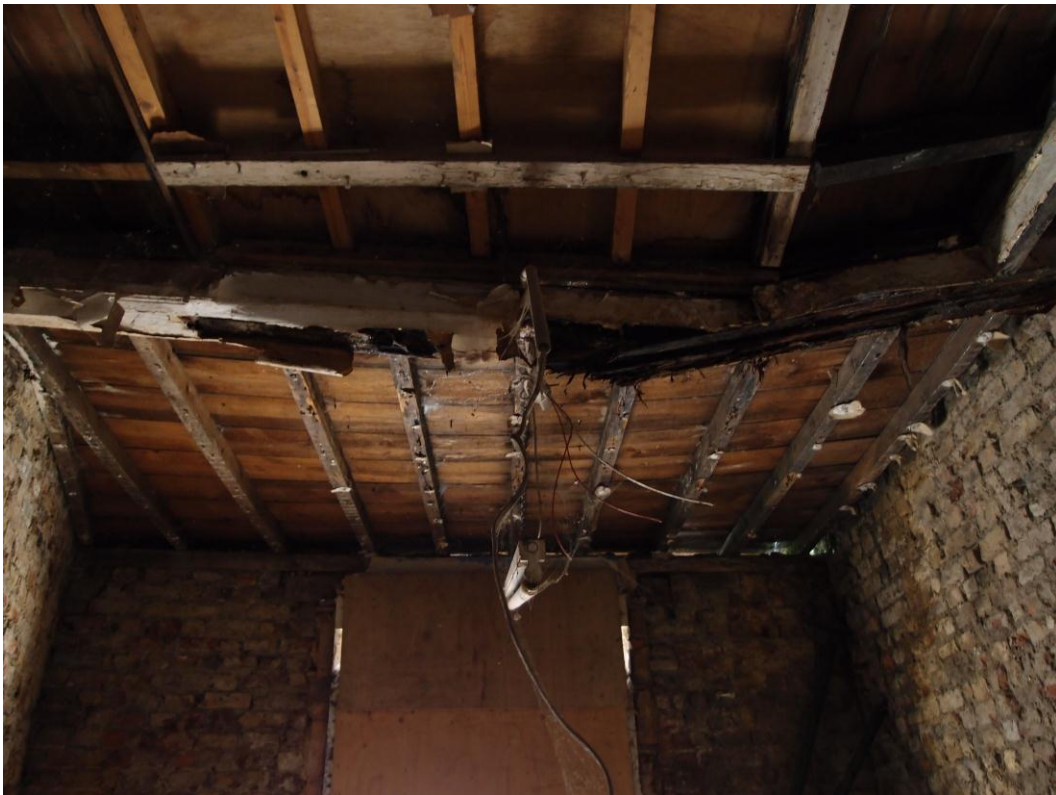
Figure 77 – Rear flat roof structure
