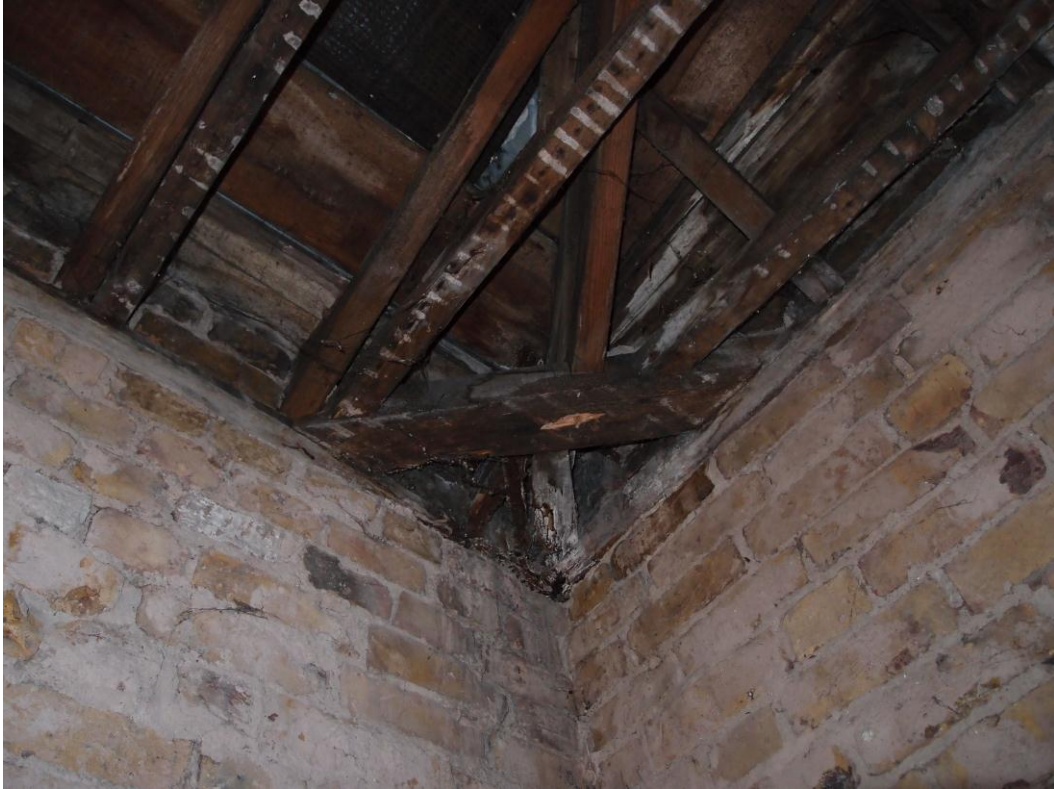
Figure 66 – Rear two story roof structure external corner hip
