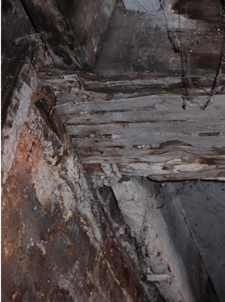
Figure 22 – First floor large beam at intersection with rear wall
