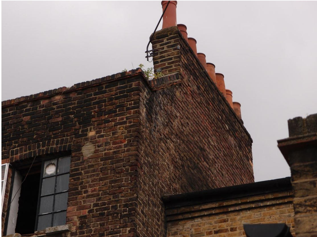
Figure 5 – Partition wall & chimney
