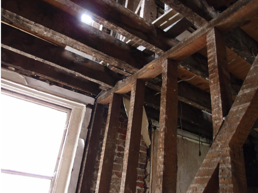
Figure 18 – Typical internal floor joists & partition
