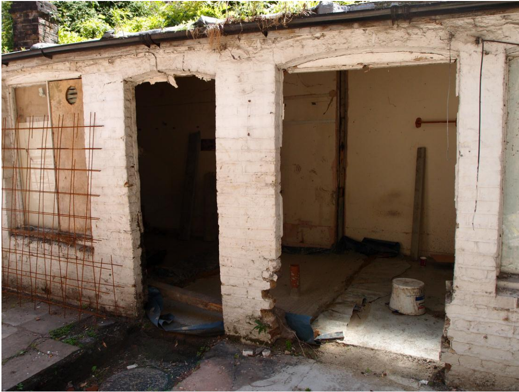
Figure 11 – Rear yard outbuilding
