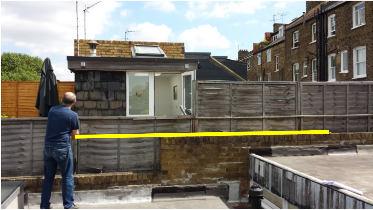
View to the north east with boundary at 76 Camden Mews (Yellow shows depth of proposed extension)
