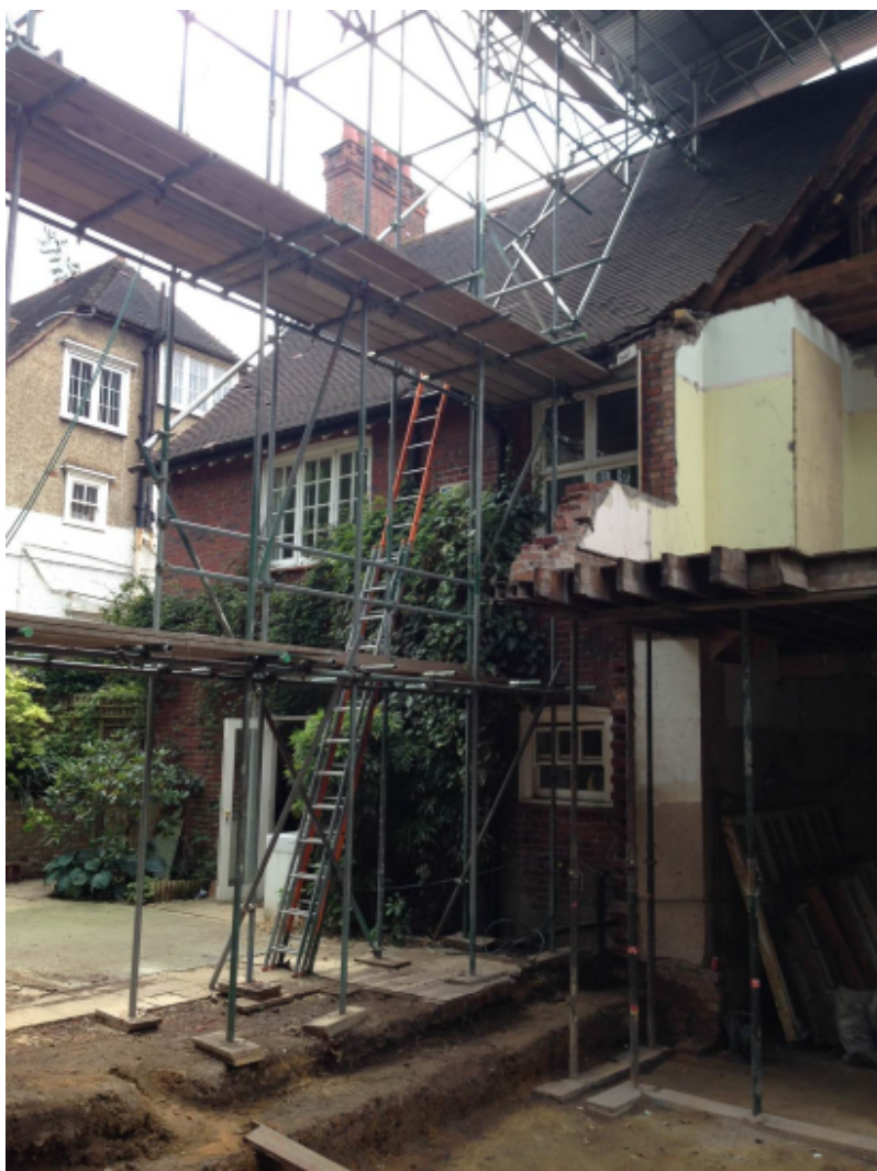
View towards rear elevation of property (showing location of proposed dormer)
