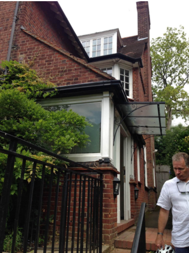
View towards front and southeast elevation
