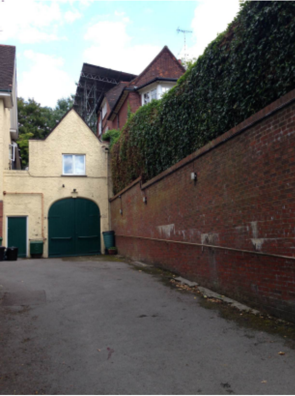
View of side elevation of property from 28 Redington Road
