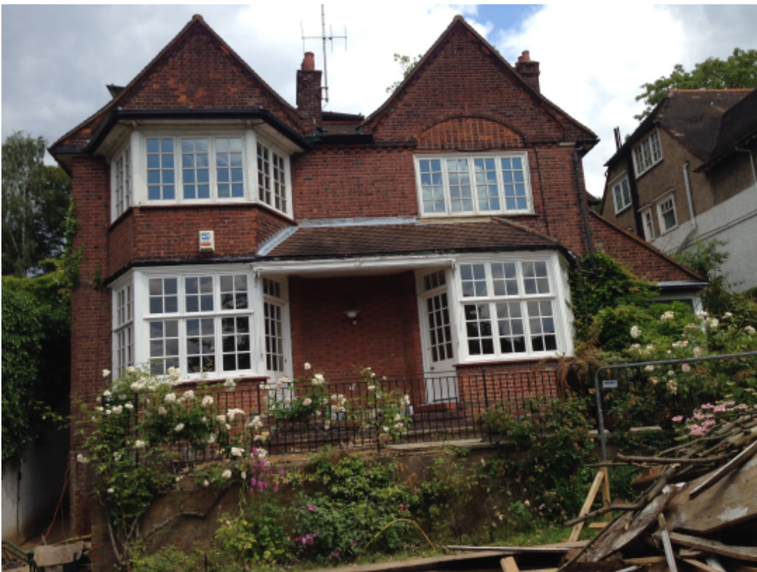
View of front of property
