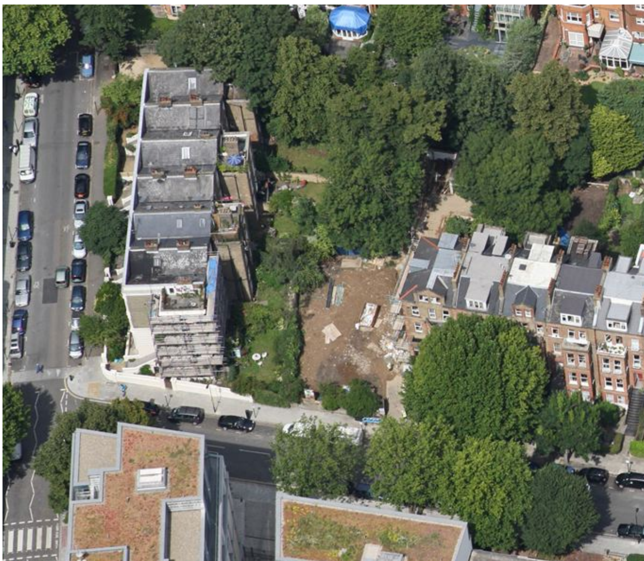
Aerial photo of site cleared prior to construction
