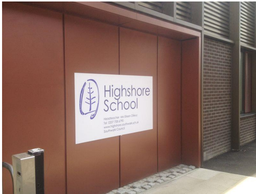
An example of quality powder coated aluminium cladding creating a pleasing palette with brickwork. This new school in Southwark Council has recently been completed.
