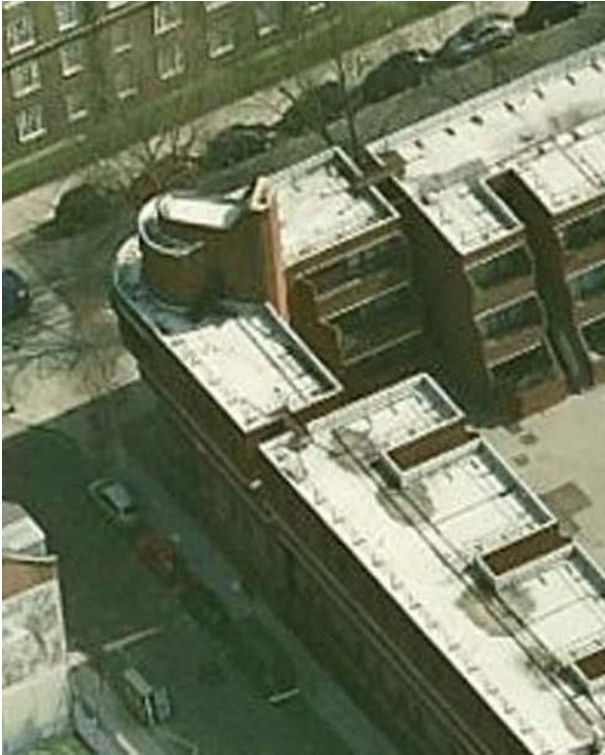
Aerial view of 87 & 88 showing the set back and towering chimney – making an extension possible in terms of scale. The photograph also shows blocks A&B as separate blocks.
