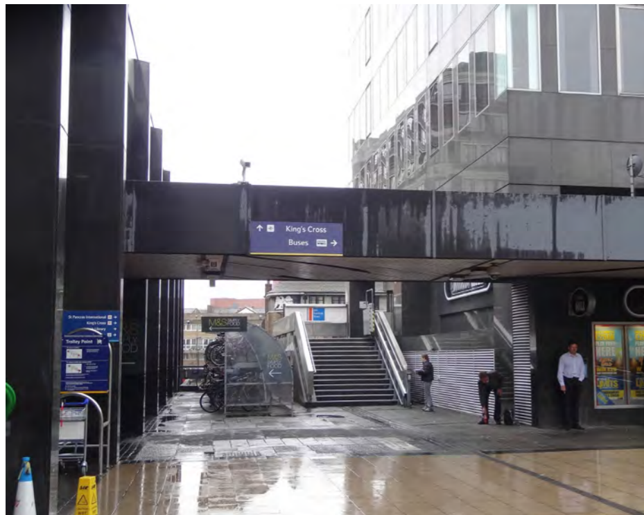
Approach from Station Square to northern entrance
