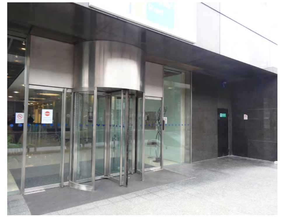
The existing northern entrance
