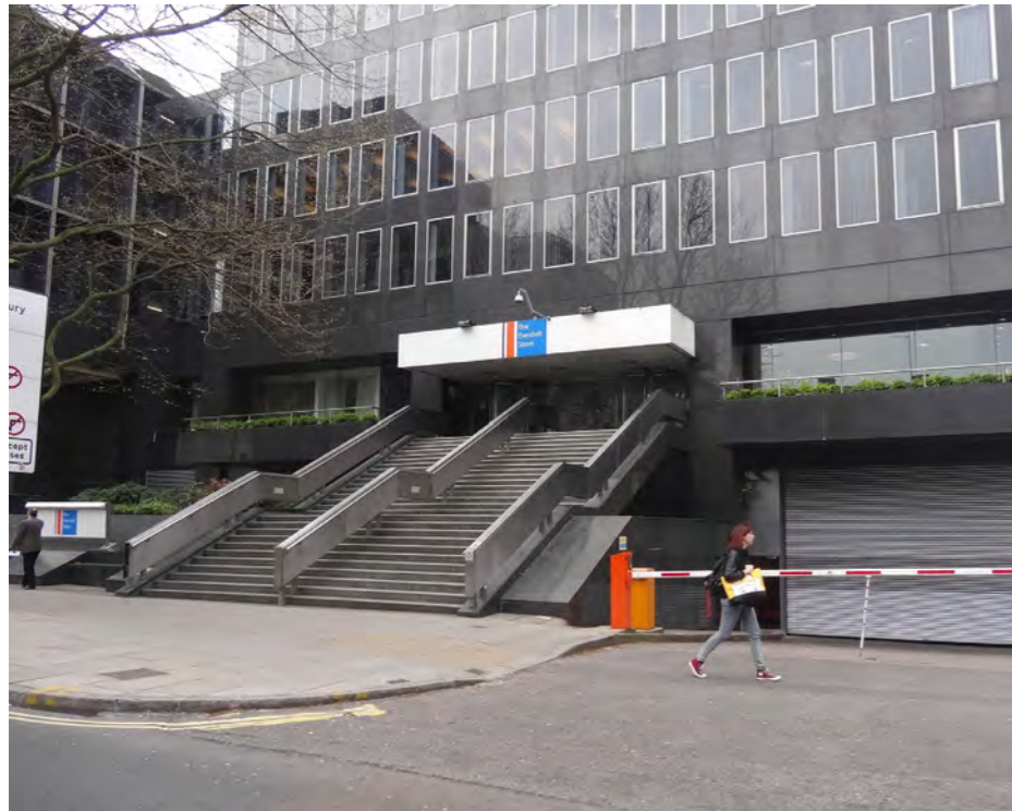
Existing eastern entrance as seen from Eversholt St
