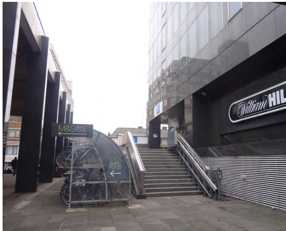
Level change from Station Square with stair lift
