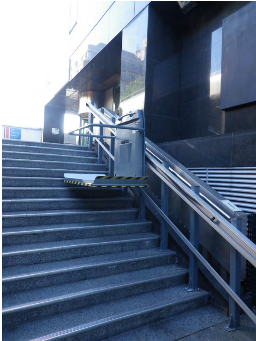
Existing entrance from Station Square with stair lift
