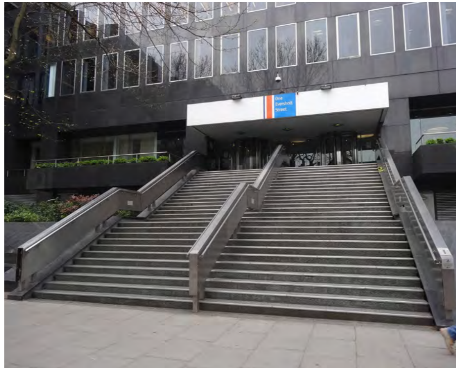
Large level change to Eversholt St entrance
