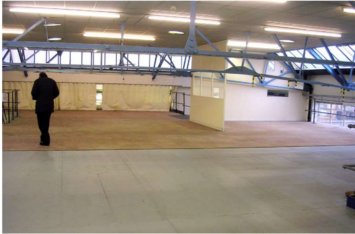
Internal views of existing commercial space (Unit 1) Mezzanine Level
