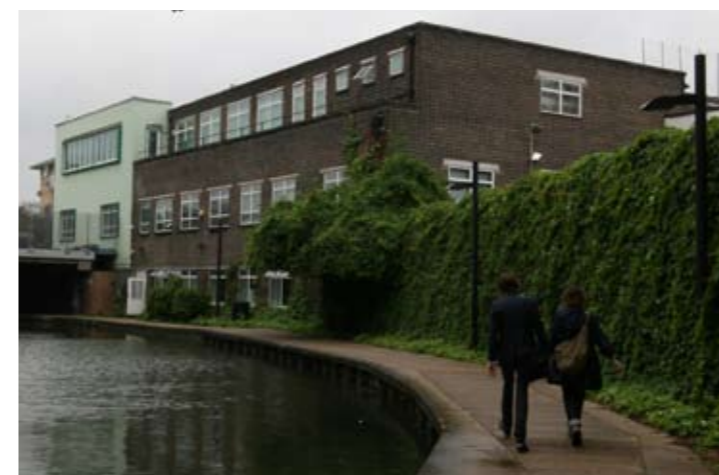
Top View along Camden Street from Shirley House Bottom View along the Regent's Canal
