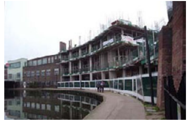
Regent's Canalside in construction
