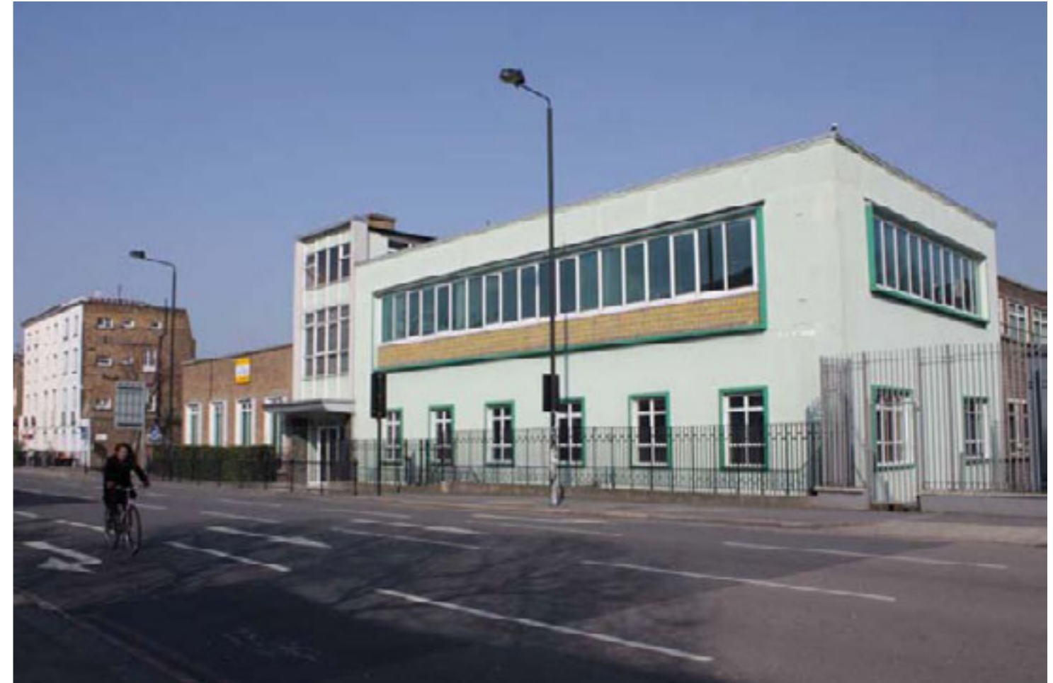
Camden Street View - Existing Building on site
