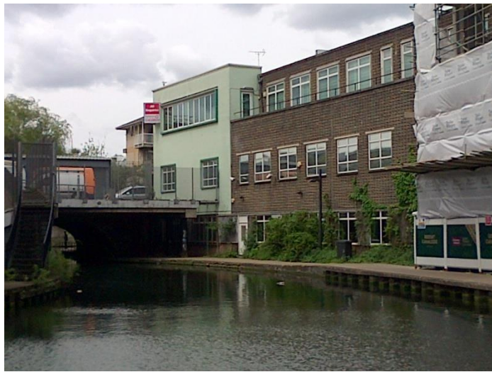
Photograph 2 Three storey office building. South-east elevation.
