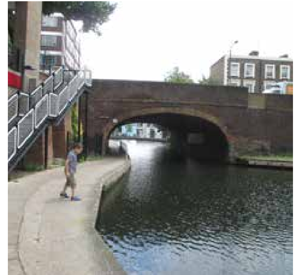
Fig. 7.2.7: North Road Bridge, looking east along the towpath.
