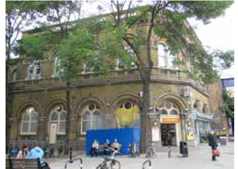
Fig. 7.2.5: E H Horne's Camden Road Station, seen from Camden Road.
