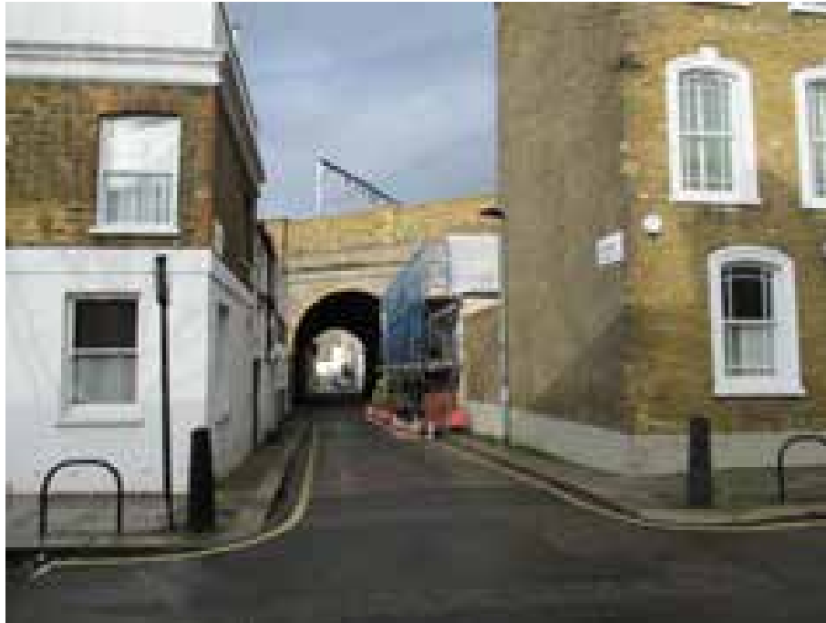
Fig. 7.1.10: View north west through Prowse Place, under the railway arches. This is view 4 of the identified important views within the conservation area.
