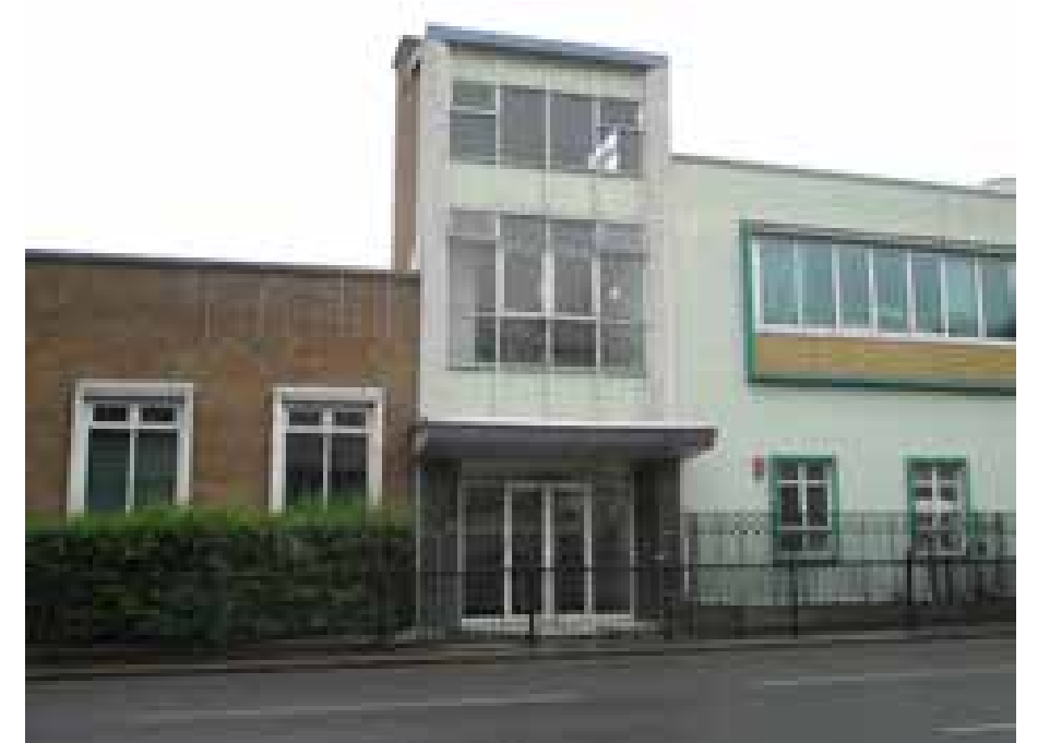
Fig. 5.7: View from Camden Street looking east, showing principal fenestration and entrance beneath canopy.
