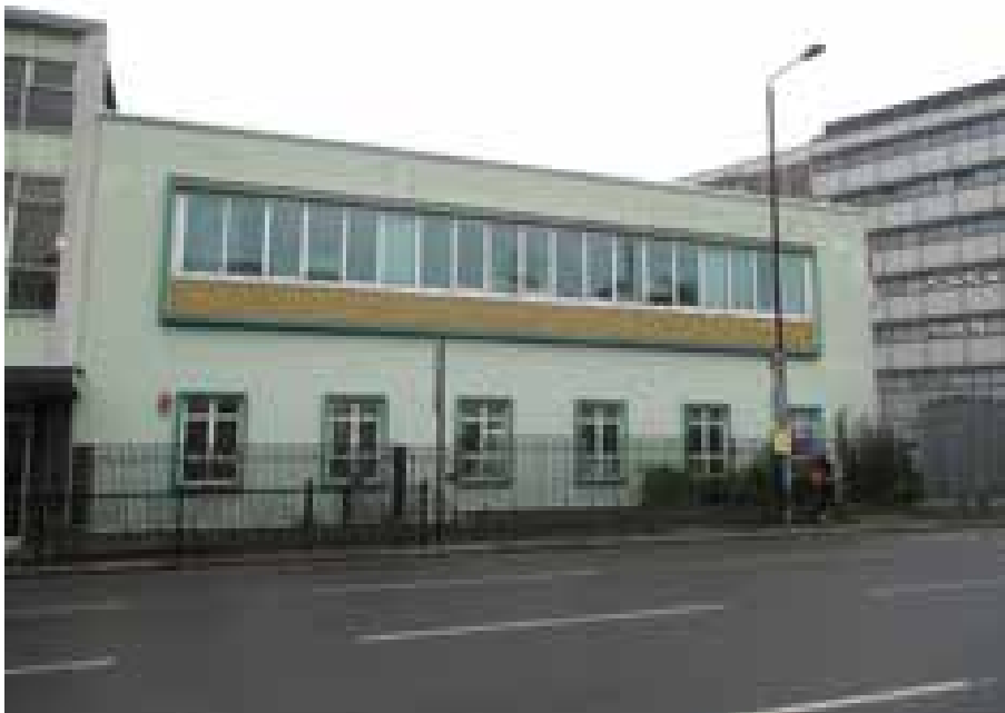
Fig. 5.8: View of the site from Camden Street looking east. Mosaic tile detailing below the first floor windows can be seen.
