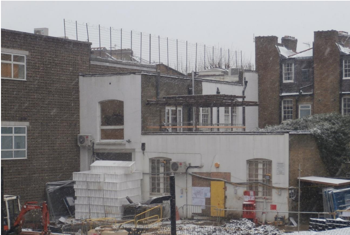
Photograph 8 Twyman House (currently under construction)
