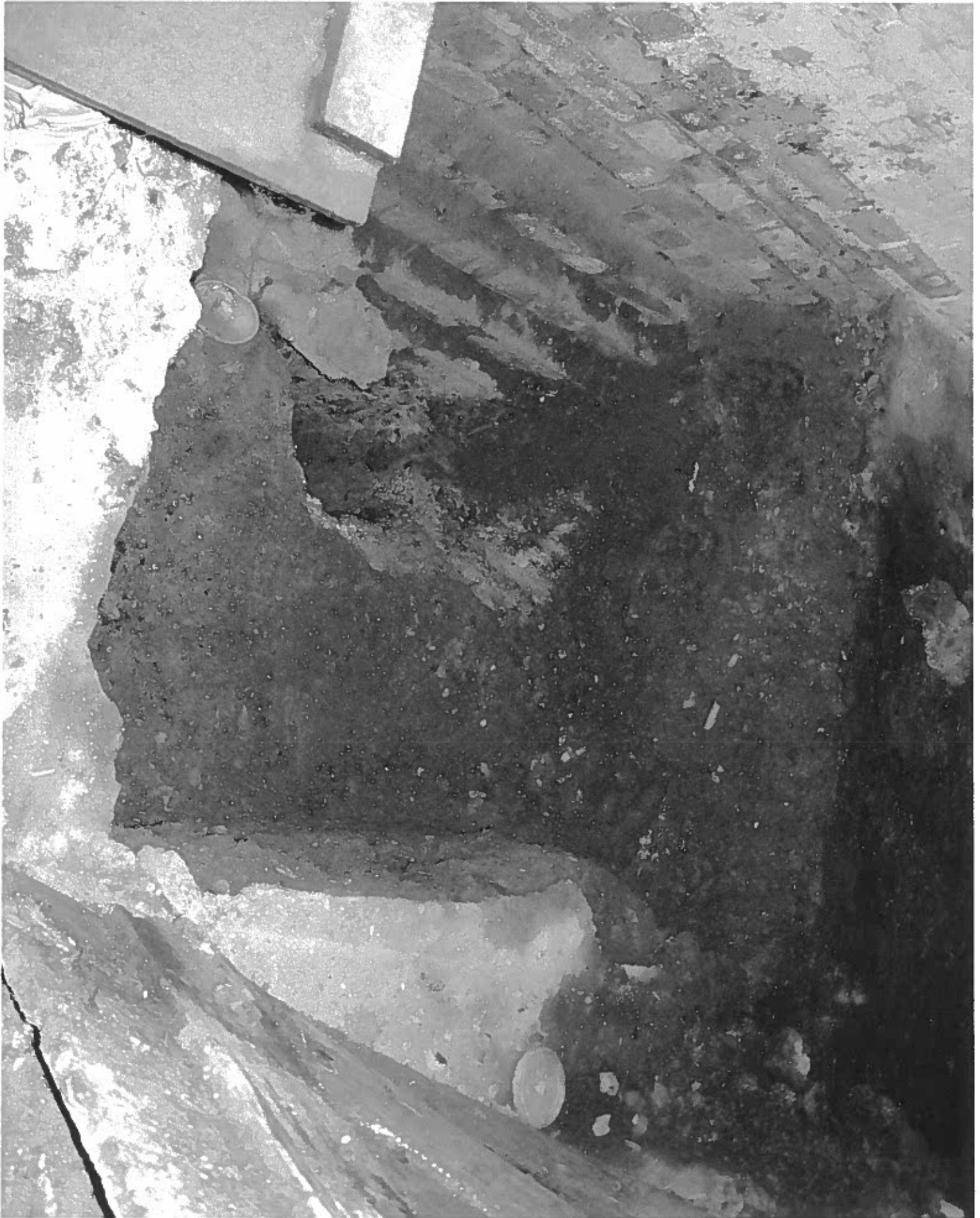
② Exposure of the foundation to L.H. Wall - Near the Staircase.
