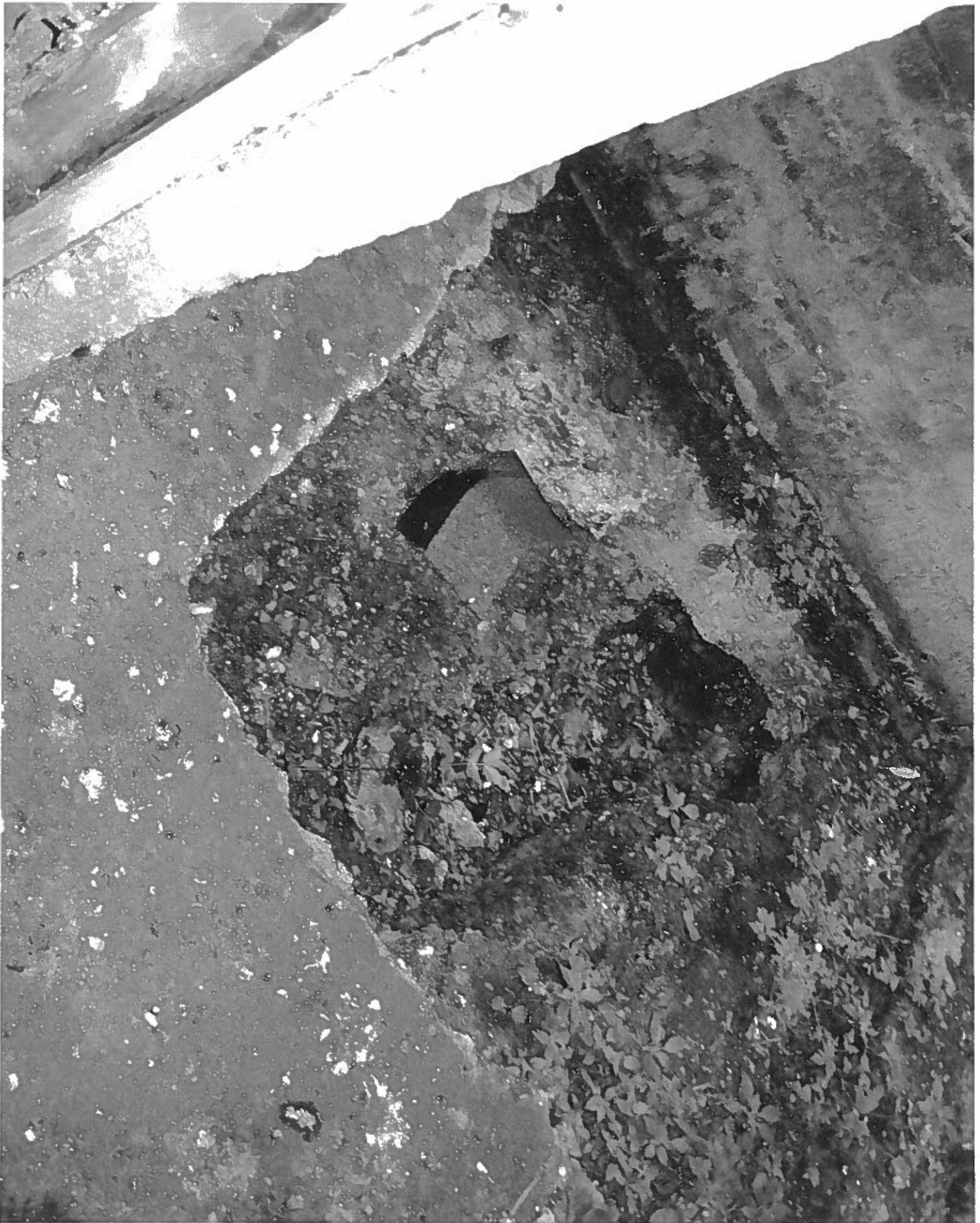
③ EXPOSURE OF THE DRAIN TO REAR YARD.
