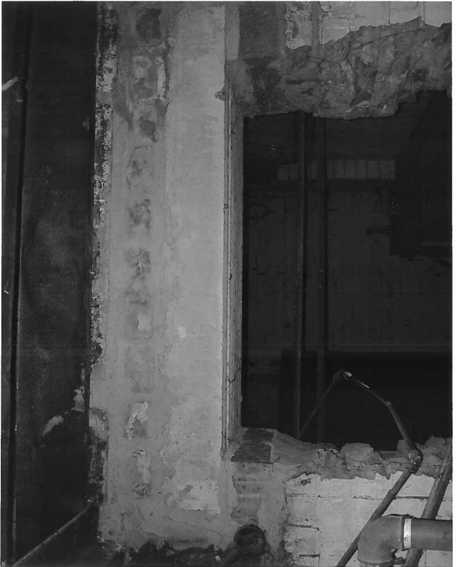
④ NEW Lintel to the Basement Bathroom Door opening.
